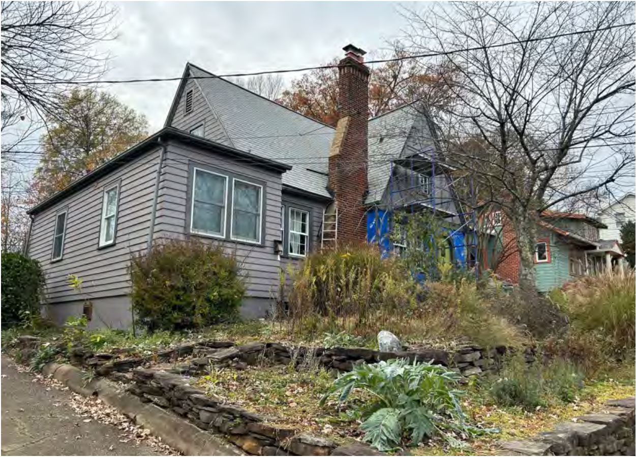
Figure 2: Front (east) and south side elevations of the subject property.
