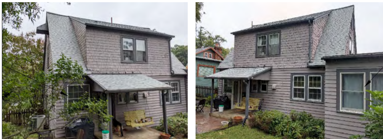
Figure 4: Existing rear elevation photographs.
