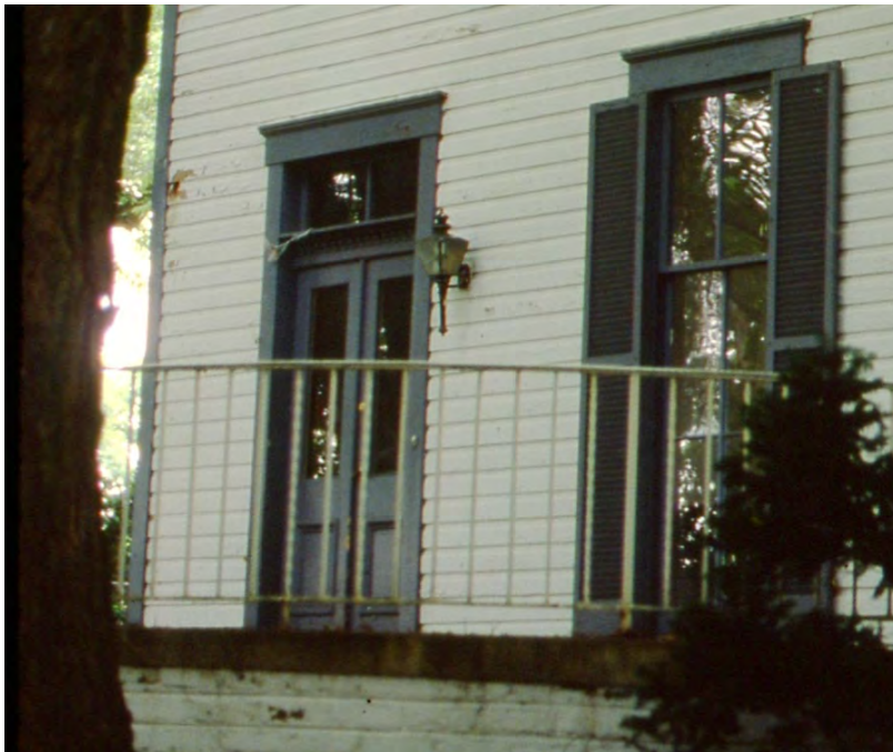
Figure 3: Undated photograph of the front doors of 15021 Rocking Spring Drive showing 3/4-length glazed panels over rectangular panels with bolection moulding below.
