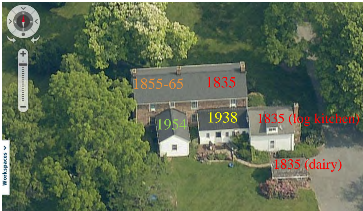
Figure 2: View of the rear elevation of the subject property, with approximate dates of construction for the various components.
