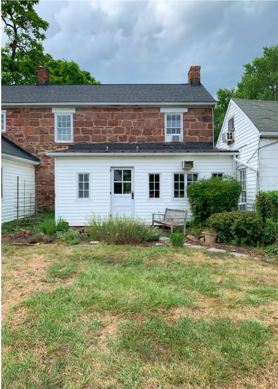
Valhala 1932 Addition South View 2024
