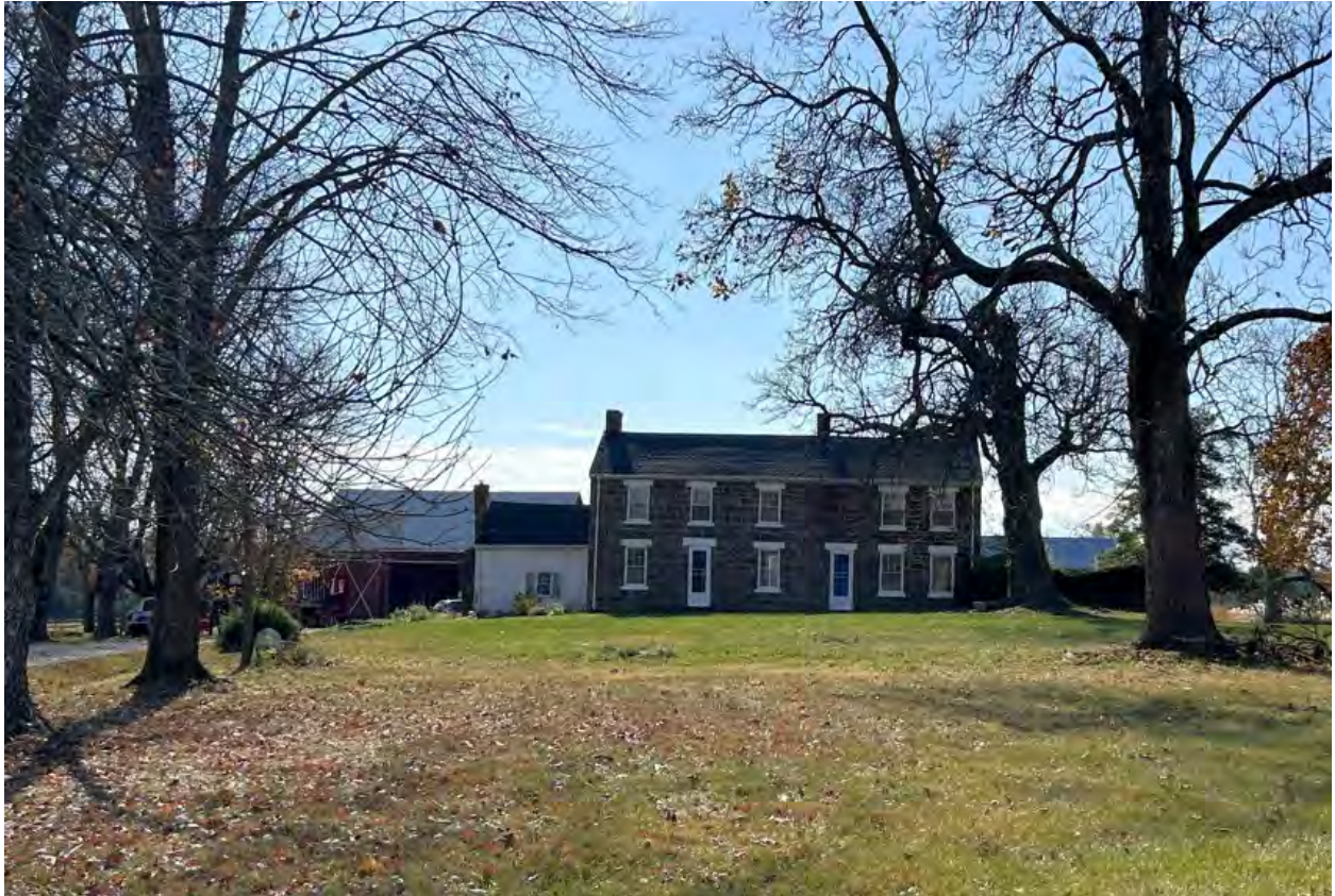
Figure 3: Front (north) elevation of the subject property.
