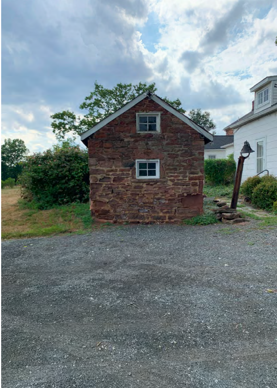
Valhala 1835 Dairy Bldg East View 2024
