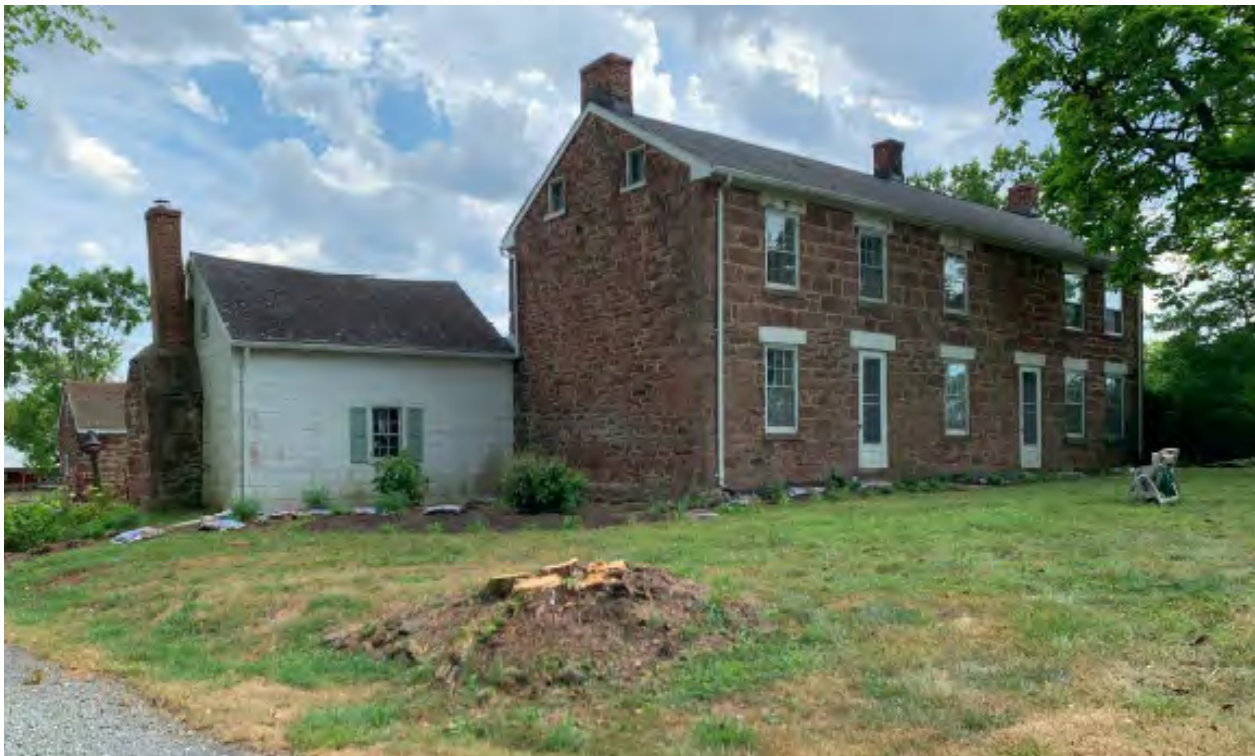
Figure 4: Front (north) and east side elevations, including the asbestos siding-clad log kitchen building on the left.
