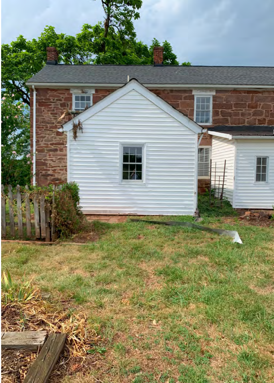
Valhala 1954 Addition South View 2024
