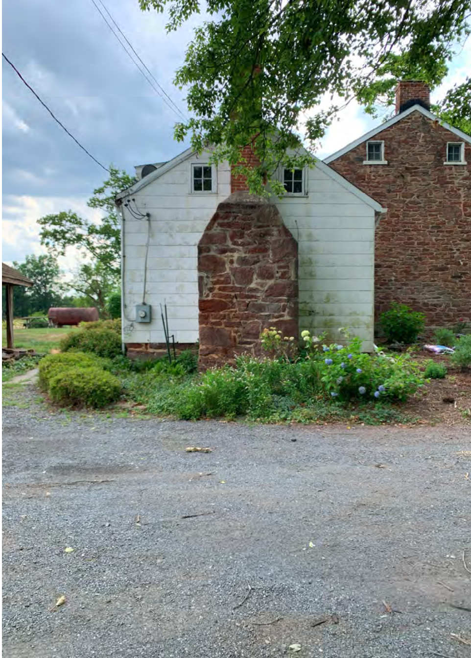
Valhala 1835 Log Bldg. East View 2024
