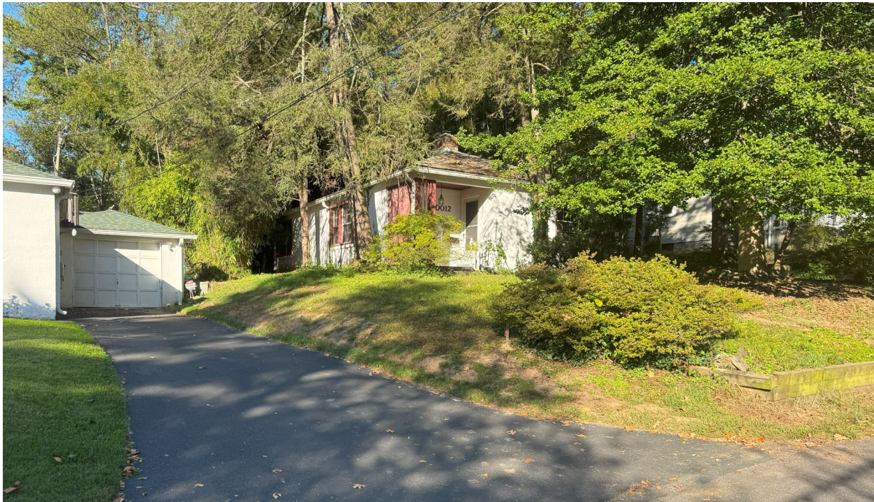
Figure 2: View showing the subject property from the south. The rearward expansion of the first floor will be visible from this perspective.
