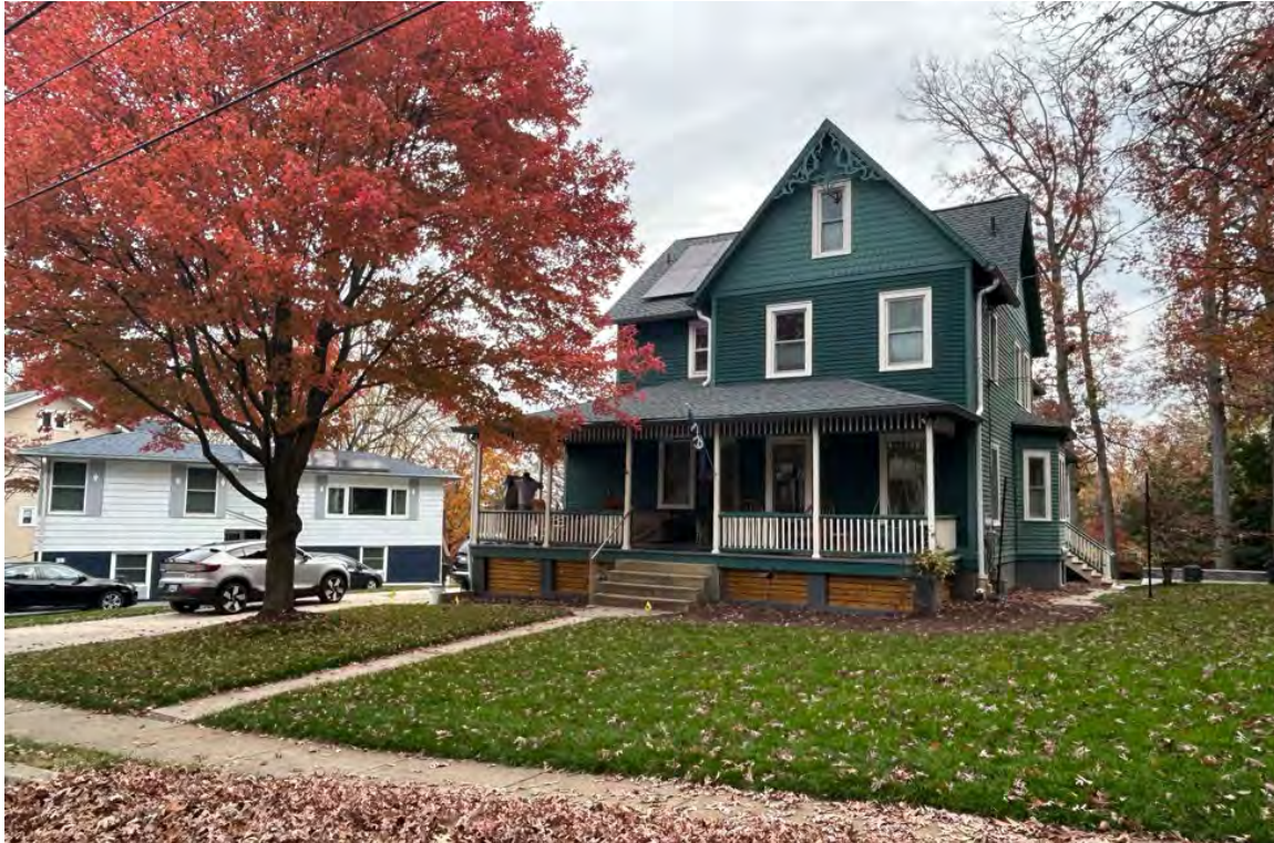
Figure 2: Front elevation of the subject property.
