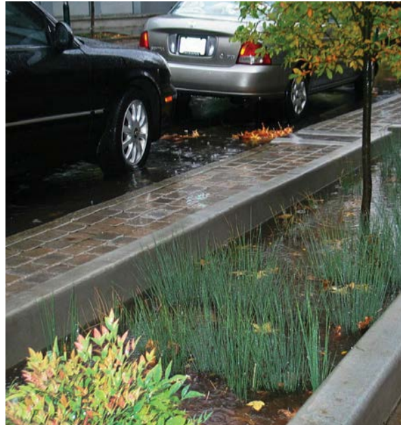
Permeable paving and curbside bioretention planters as evaporative cooling elements
