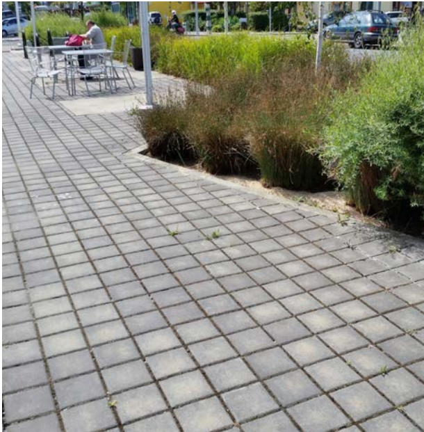
Permeable paving and curbside bioretention planters as evaporative cooling elements
