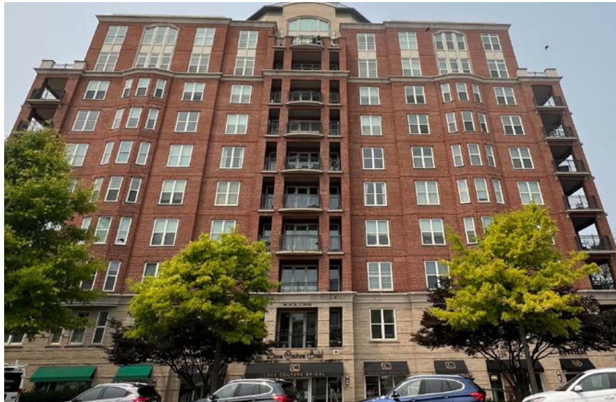
Figure 39: Multi-family apartment with ground floor retail on Main Street at Park Potomac
