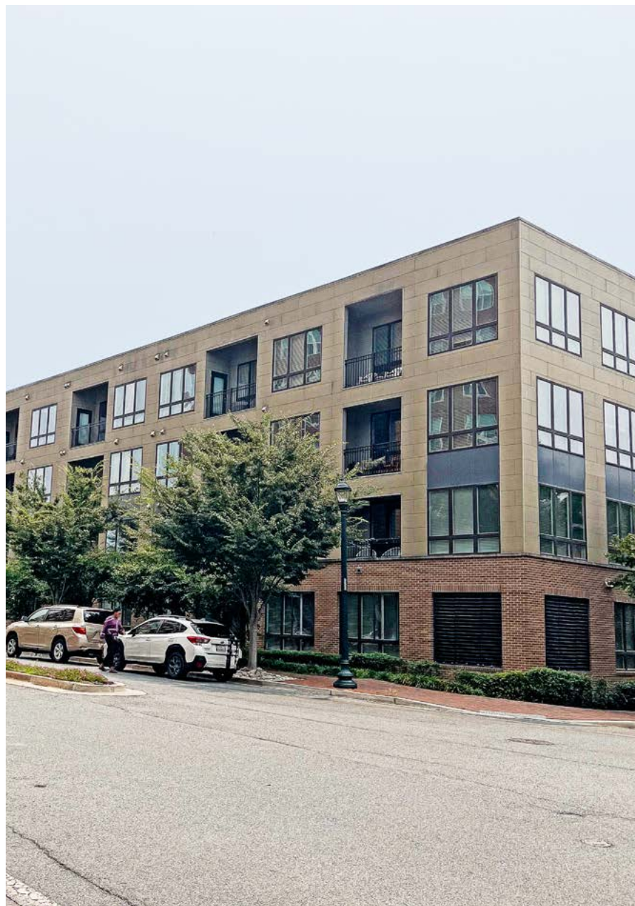
Figure 43: Multi-family apartments in residential neighborhood of Park Potomac
