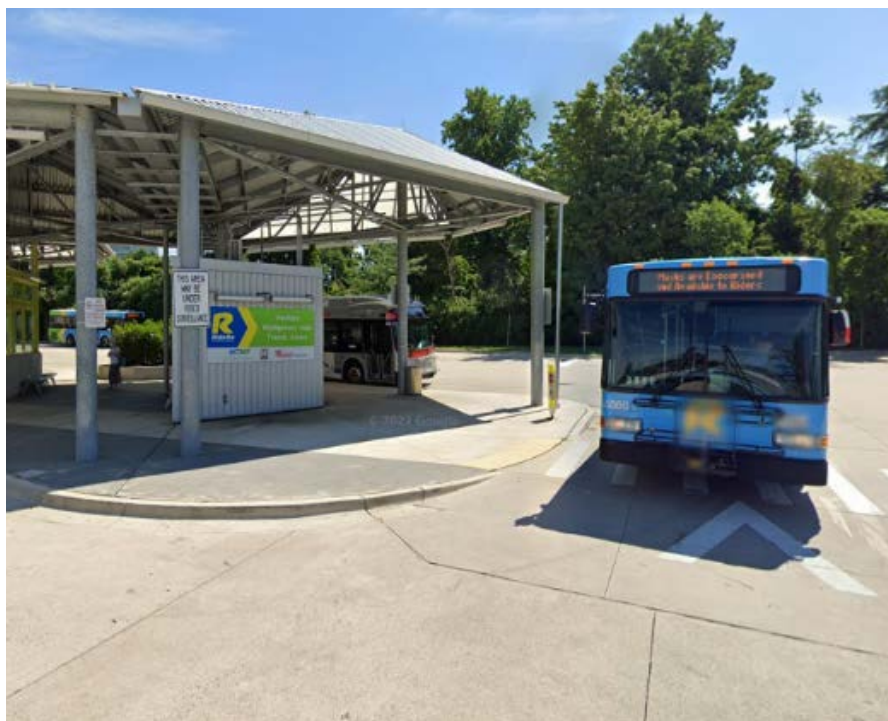
Figure 58: Montgomery Mall Transit Center
