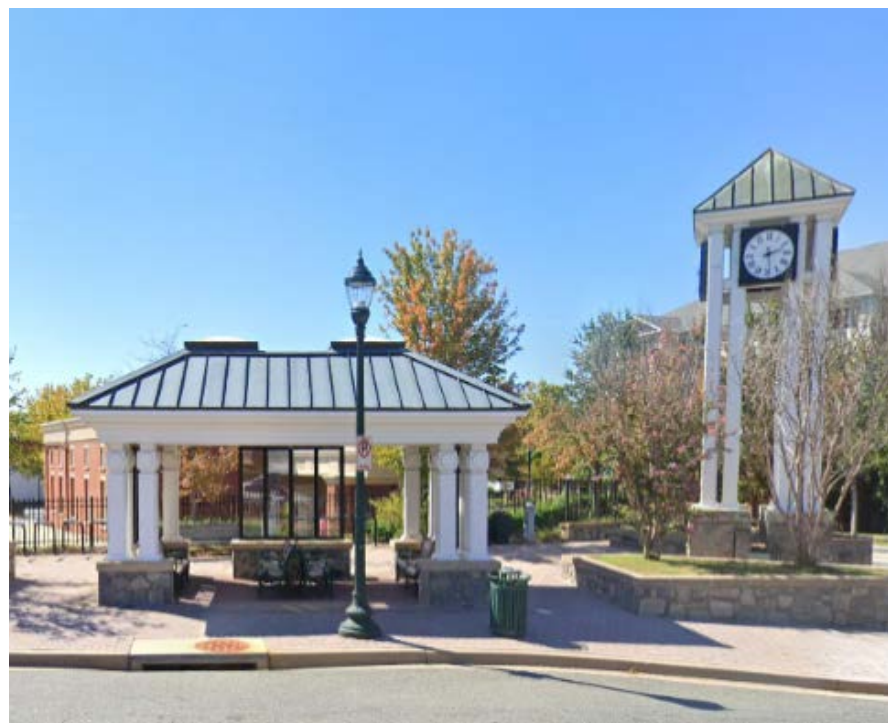
Figure 59: Trville Development Transit Center
