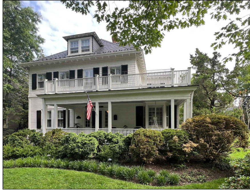
A1 A12 NTS EXISTING EXTERIOR VIEW - FRONT
