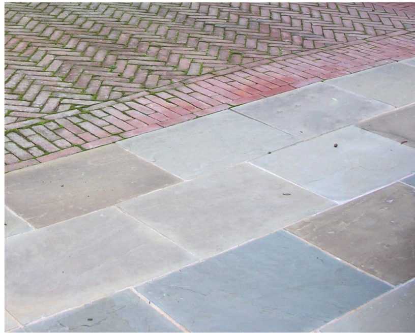
PROPOSED BLUESTONE AND BRICK PAVING
