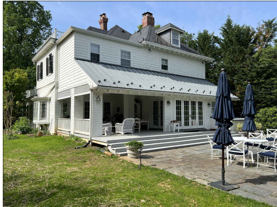
B1 A12 NTS EXISTING EXTERIOR VIEW - REAR
