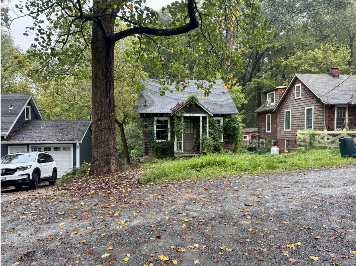
Figure 2: The subject property is a small cottage near the north end of the Hawkins Lane Historic District.
