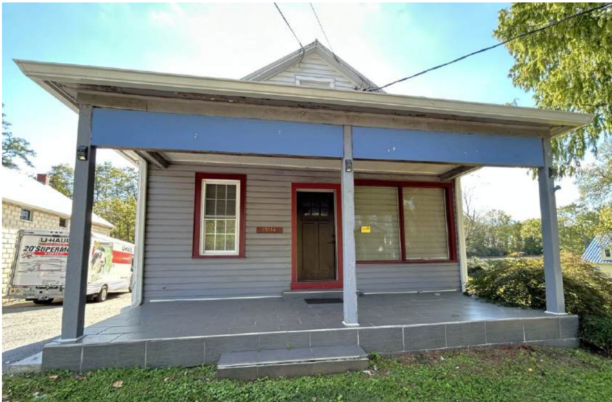
Figure 10: Front elevation, October 2024 (Historic Preservation Office).
