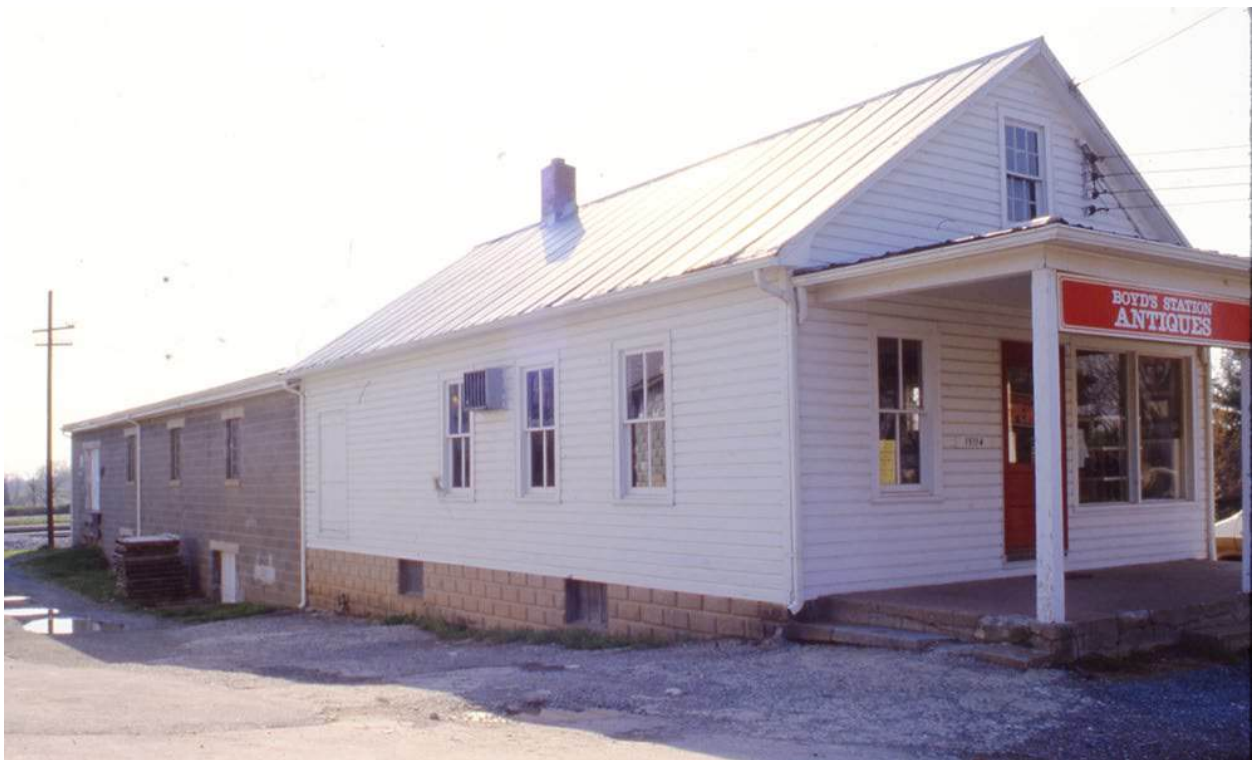
Figure 3: 15114 Barnesville Road, front (north) and east side elevations, 1986 (MCAtlas).
