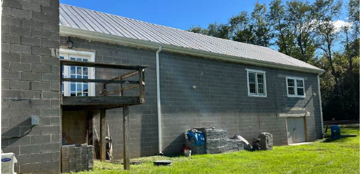
Figure 13: West elevation of the rear CMU addition, October 2024 (Historic Preservation Office). Recent window alterations have been undertaken, and additional alterations are proposed.
