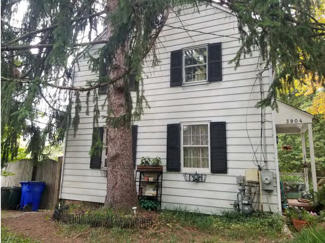
North side of the house
