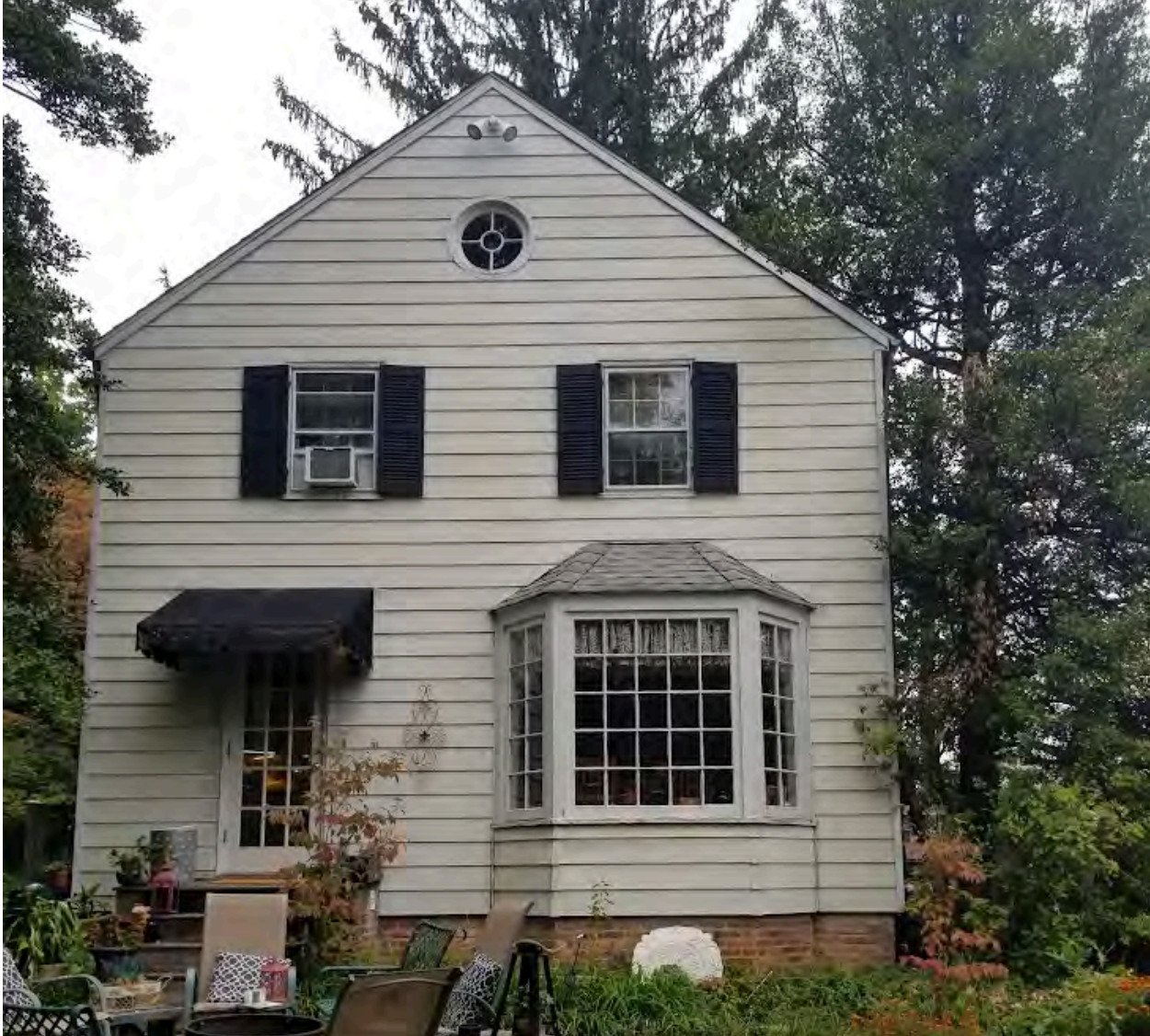
South side of the house
