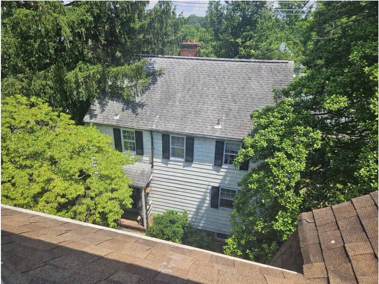
Western face of roof as viewed from 2nd floor window of 3906 Washington Street
