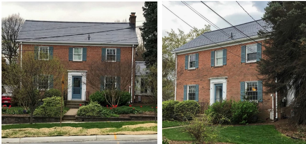
Figure 7: 1946 Seminary Rd., Silver Spring (across from the fire station) is one of the first solar shingle installations in the county.
