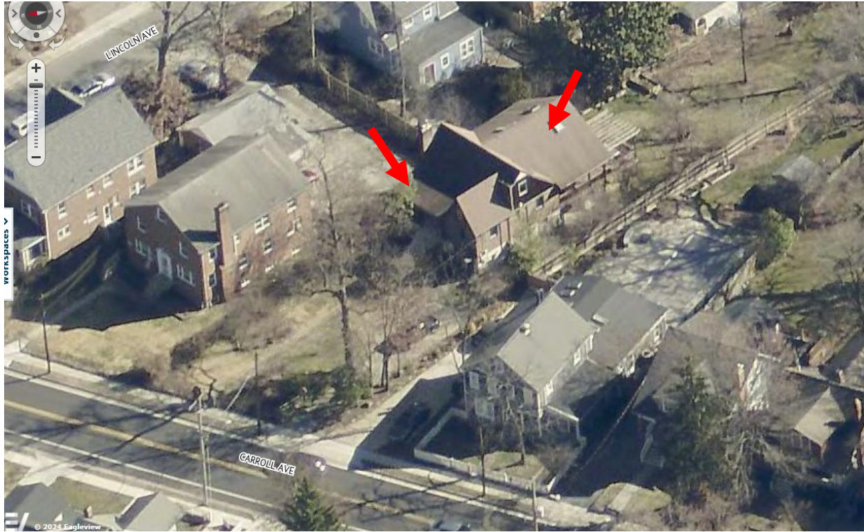
Figure 6: Birds-eye view looking east towards the property (February 2024, ConnectExplorer). Red arrows point to the array locations.
