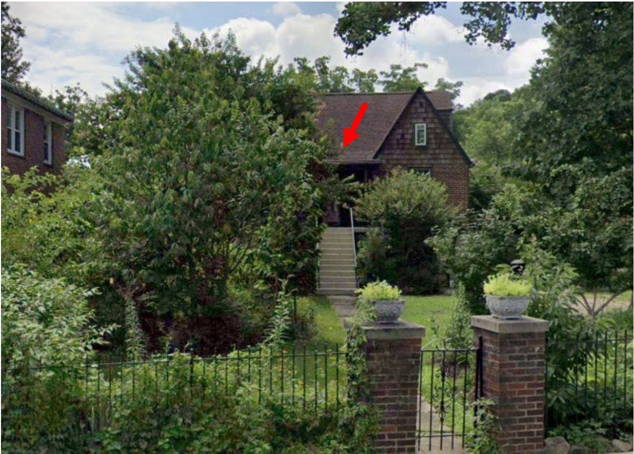
Figure 5: The front (northwest) elevation of 7425 Carroll Avenue (Google Streetview, July 2022). A red arrow points to the front panel location on the low-slope porch roof.
