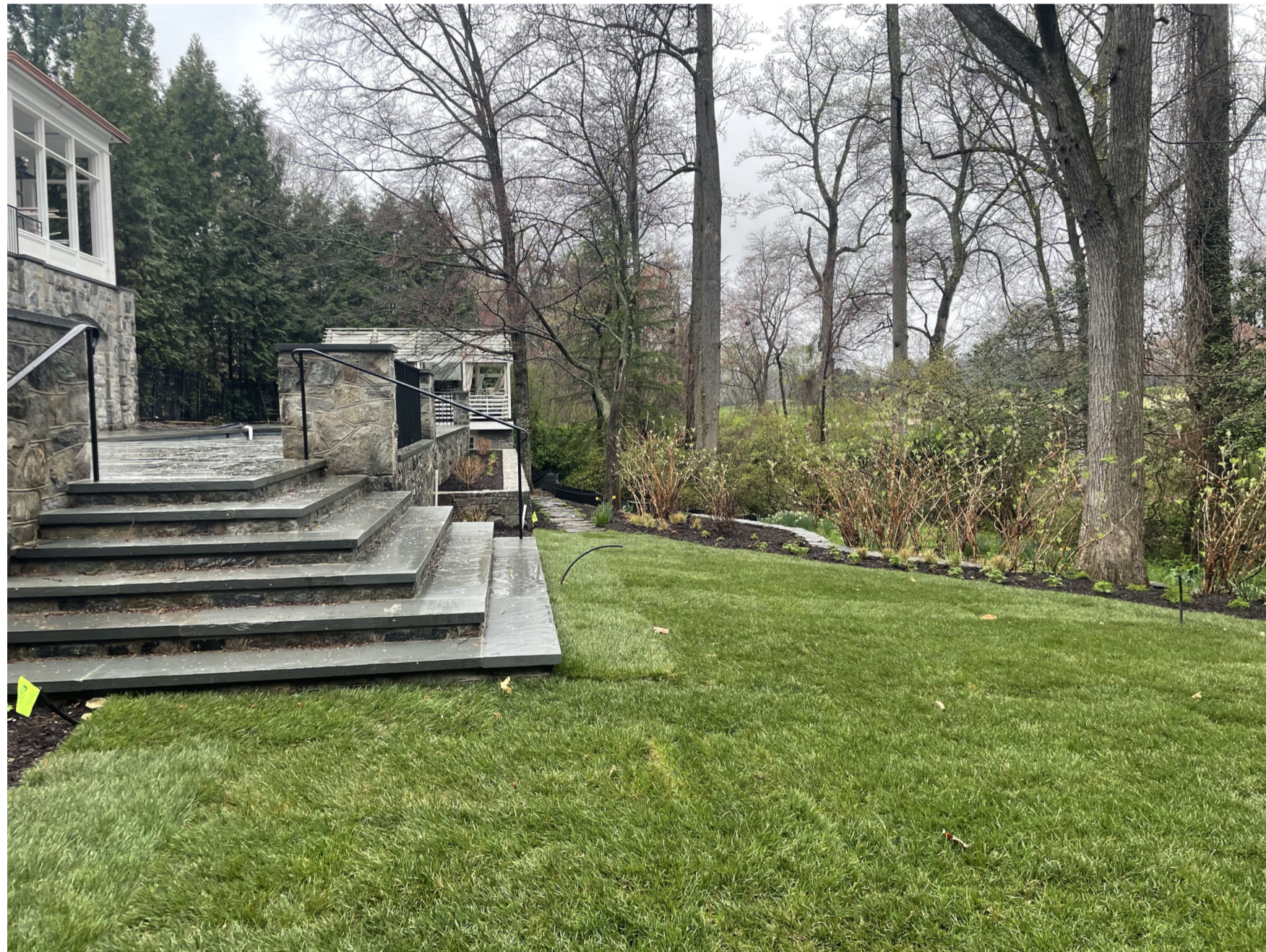
EXISTING STAIRS TO LOWER LAWN
