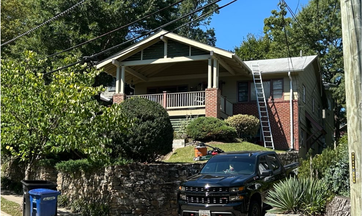
Figure 2: The front (southeast) elevation of 34 Columbia Ave. from the sidewalk in front of the house, September 2024 (Historic Preservation Office). The prominent front porch was approved by the HPC in 2011.
