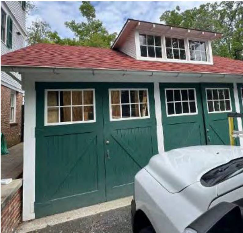
Front of detached Structure
