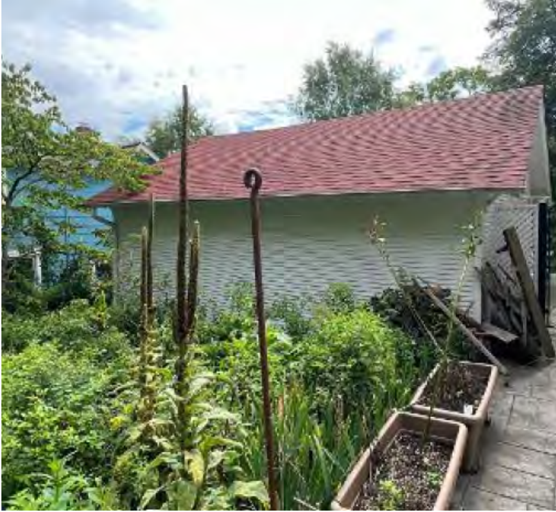
Back Side of detached structure
