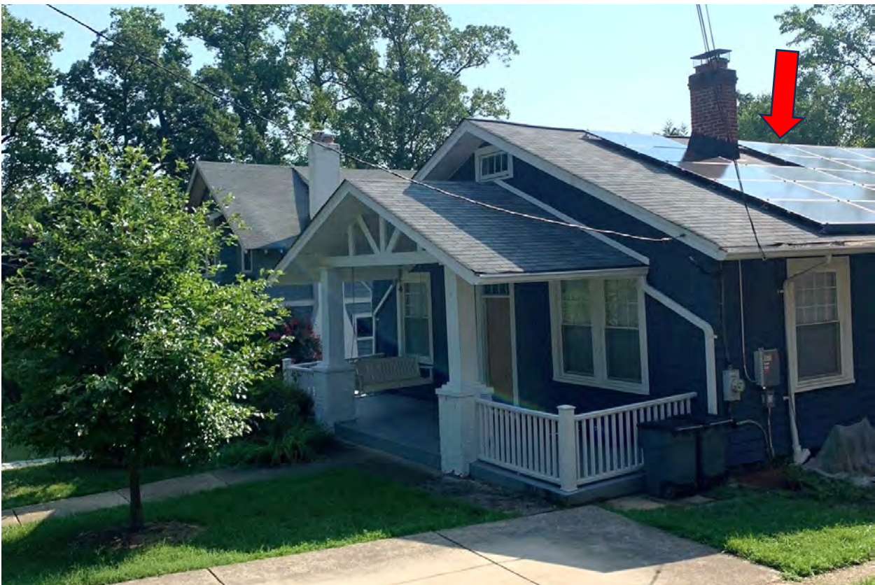
Figure 13: The HPC approved solar panels on the nearby Contributing resource at 7207 Willow Avenue (indicated with a red arrow) at the November 15, 2023, meeting.
