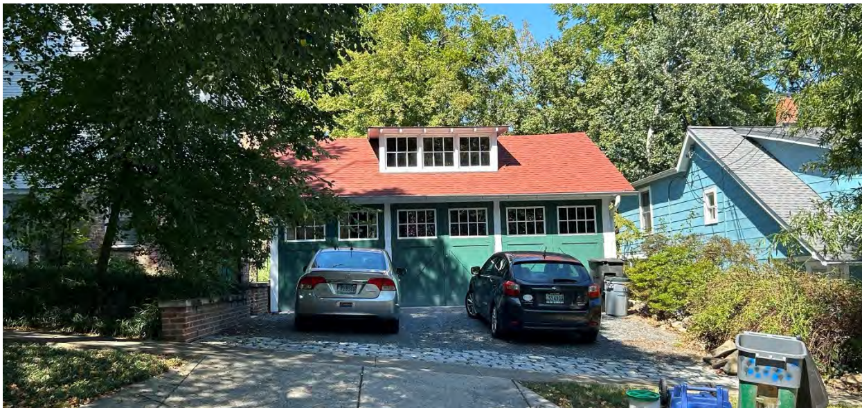
Figure 3: The southeast elevation of the rear garage, which faces Willow Avenue, September 2024 (Historic Preservation Office).
