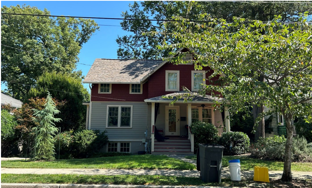
Figure 3: The front (west) elevation of 28 Hickory Avenue, September 2024 (Historic Preservation Office).
