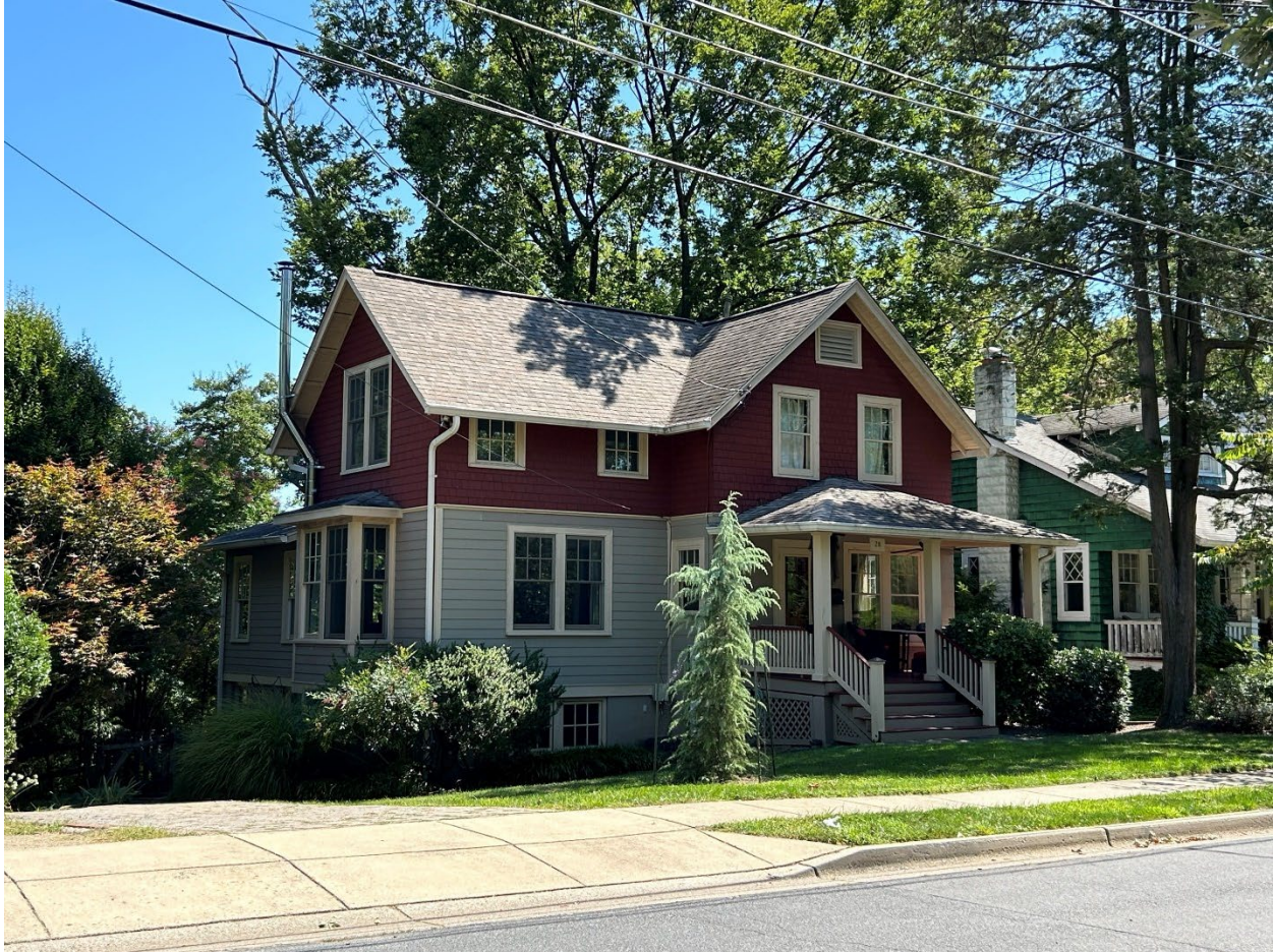
Figure 2: The front (west) elevation of 28 Hickory Avenue, September 2024 (Historic Preservation Office).
