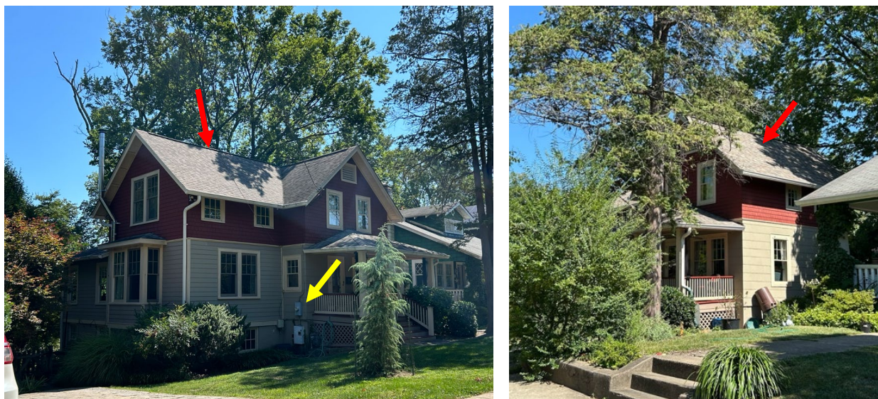
Figure 6: Visibility of panel locations (red arrows) and associated equipment (yellow arrow).
