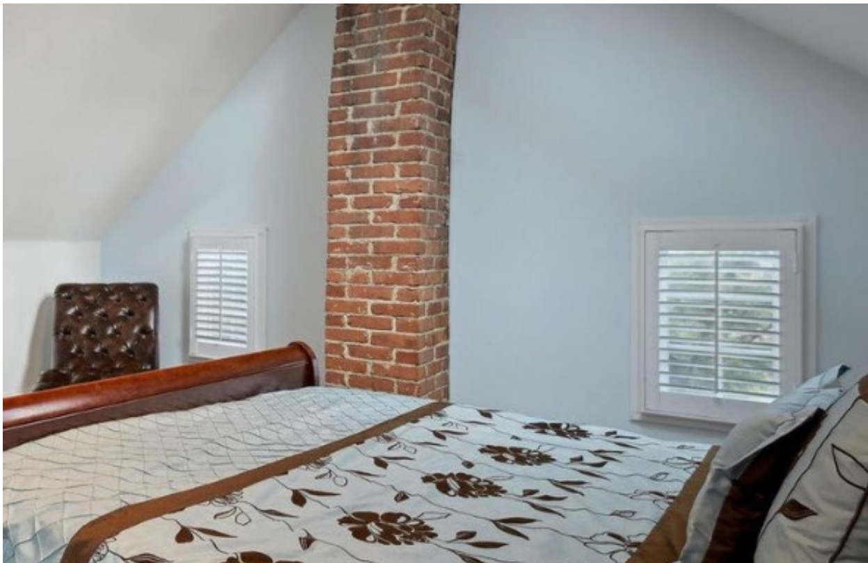
Figure 12: Interior photographs of the third-floor, east-facing windows prior to alterations (c. Spring 2024, MLS via Redfin). The property was listed for sale in March 2024 and sold in May 2024.
