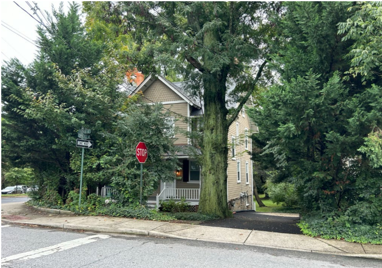
Figure 2: The front elevation of the subject property at 3820 Warner Street, September 2024 (Historic Preservation Office).
