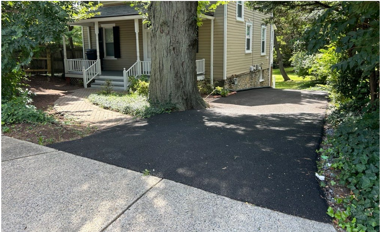
Figure 5: View of the full extent of the newly-paved driveway, September 2024 (Historic Preservation Office).
