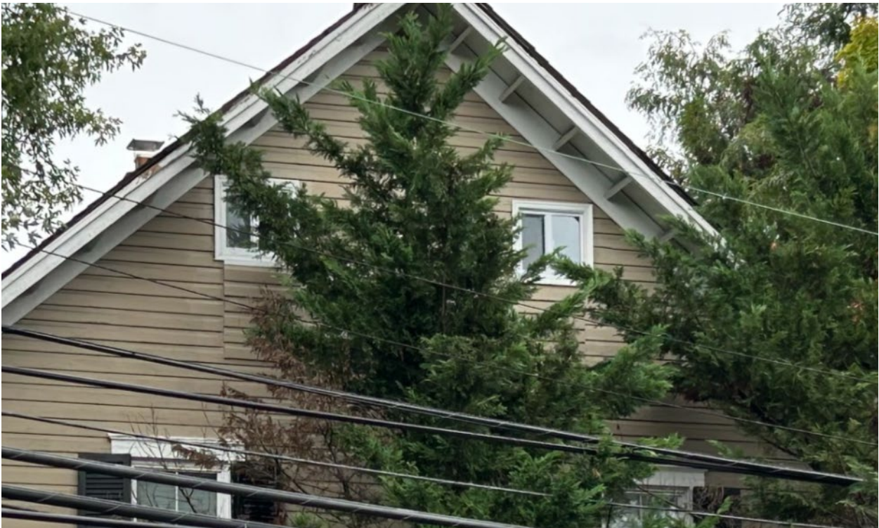
Figure 10: The third-floor, east-facing windows after alterations (September 2024, Historic Preservation Office).
