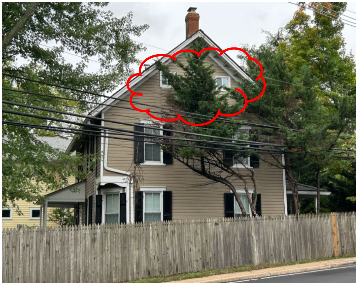
Figure 7: The east elevation of 3820 Warner Street, from Connecticut Avenue (September 2024, Historic Preservation Office). The altered third-floor windows are circled in red.
