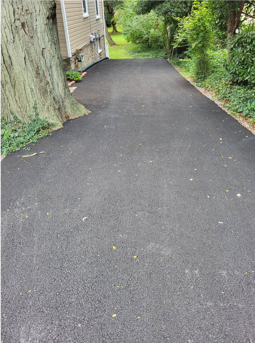
Figure 4: Newly installed driveway tree on left.
