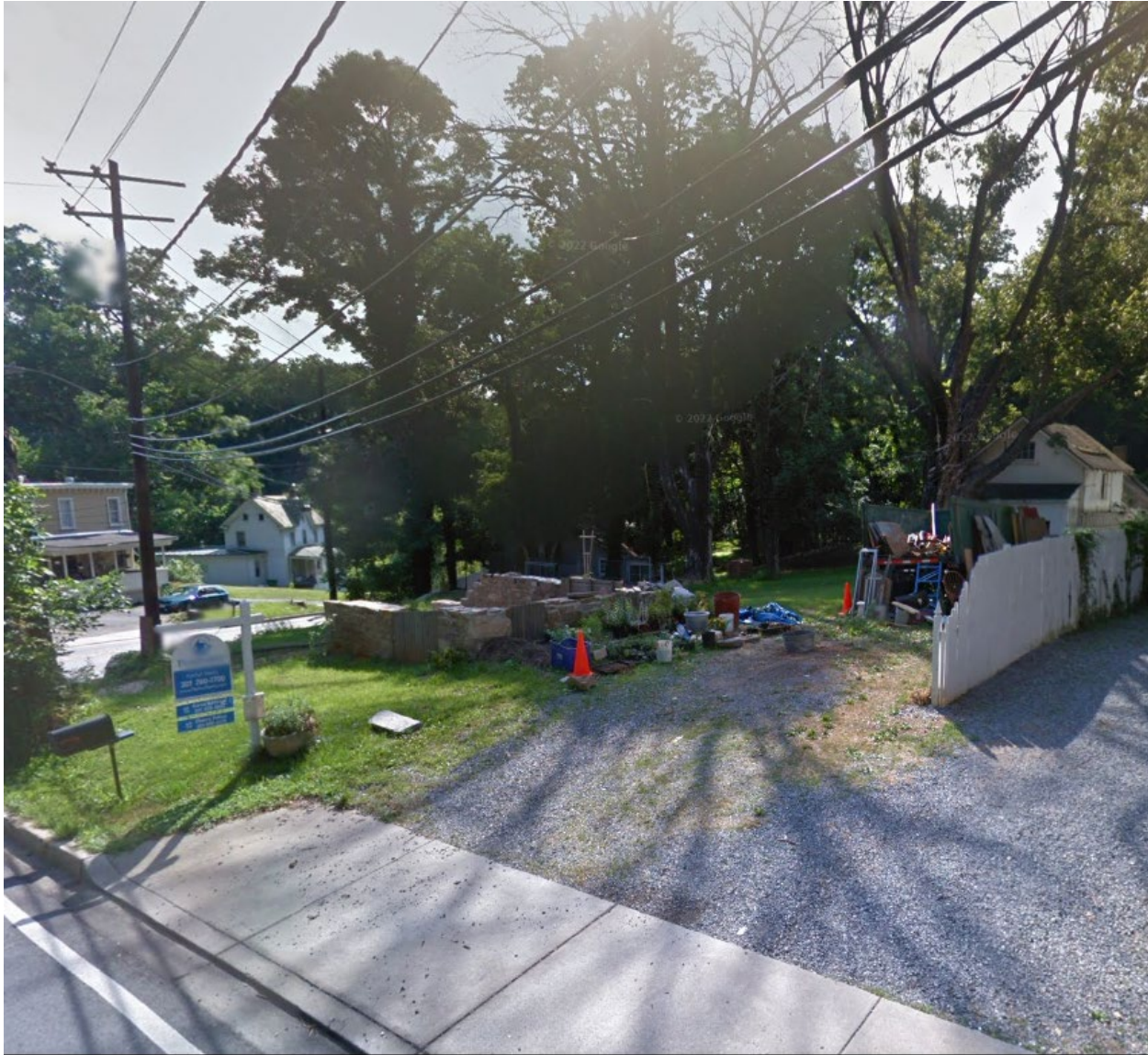
Figure 3: Streetview image after the demolition of the main house from Market Street. The stone foundation remains extant. The shed is visible to the far right. (Google streetview from 2012)
