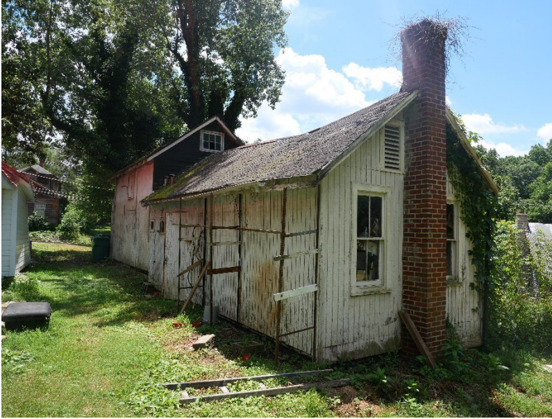
Figure 8: Rear view of the outbuilding proposed for removal. (Historic Preservation Office, 2024)
