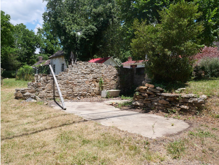
Figure 4: Extant basement foundation walls viewed from Market Street. (Historic Preservation Office, June 2024)
