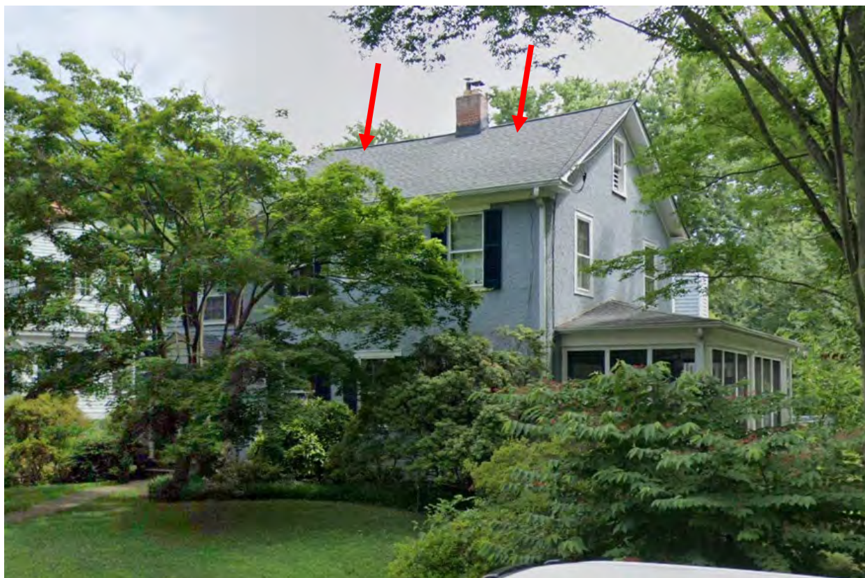
Figure 5: Front elevation of 2929 Washington Avenue (Google Streetview, July 2022).
