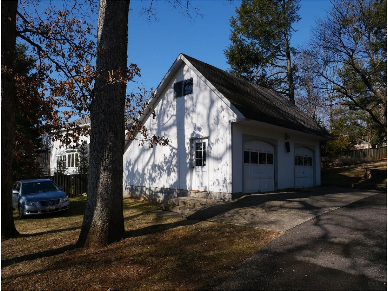
Figure 13: View of the 1989 garage (looking northwest), 2022. Source: Historic Preservation Office, Montgomery Planning.
