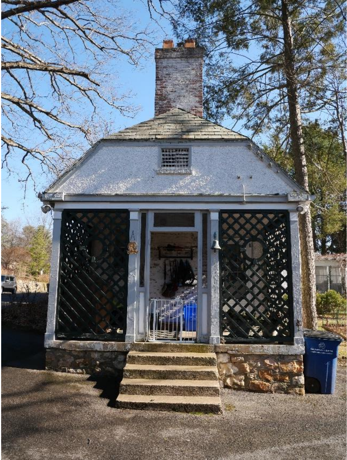
Figure 4: View of the west elevation of the 1930 kitchen addition, 2022. Source: Historic Preservation Office, Montgomery Planning.
