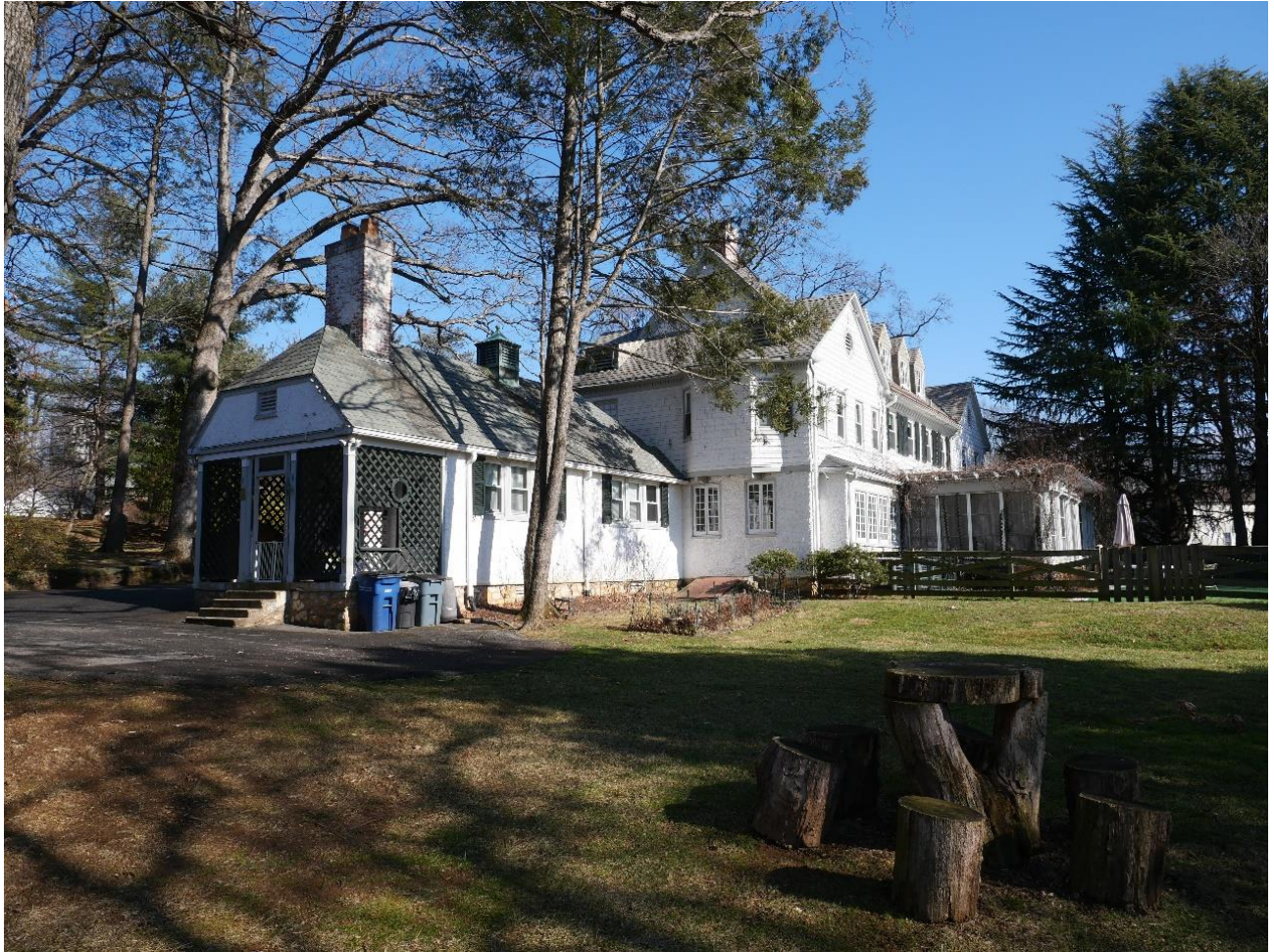
Figure 5: Axial view of the west and south elevations of the 1930 kitchen addition and 1901 home (looking northeast), 2022.
