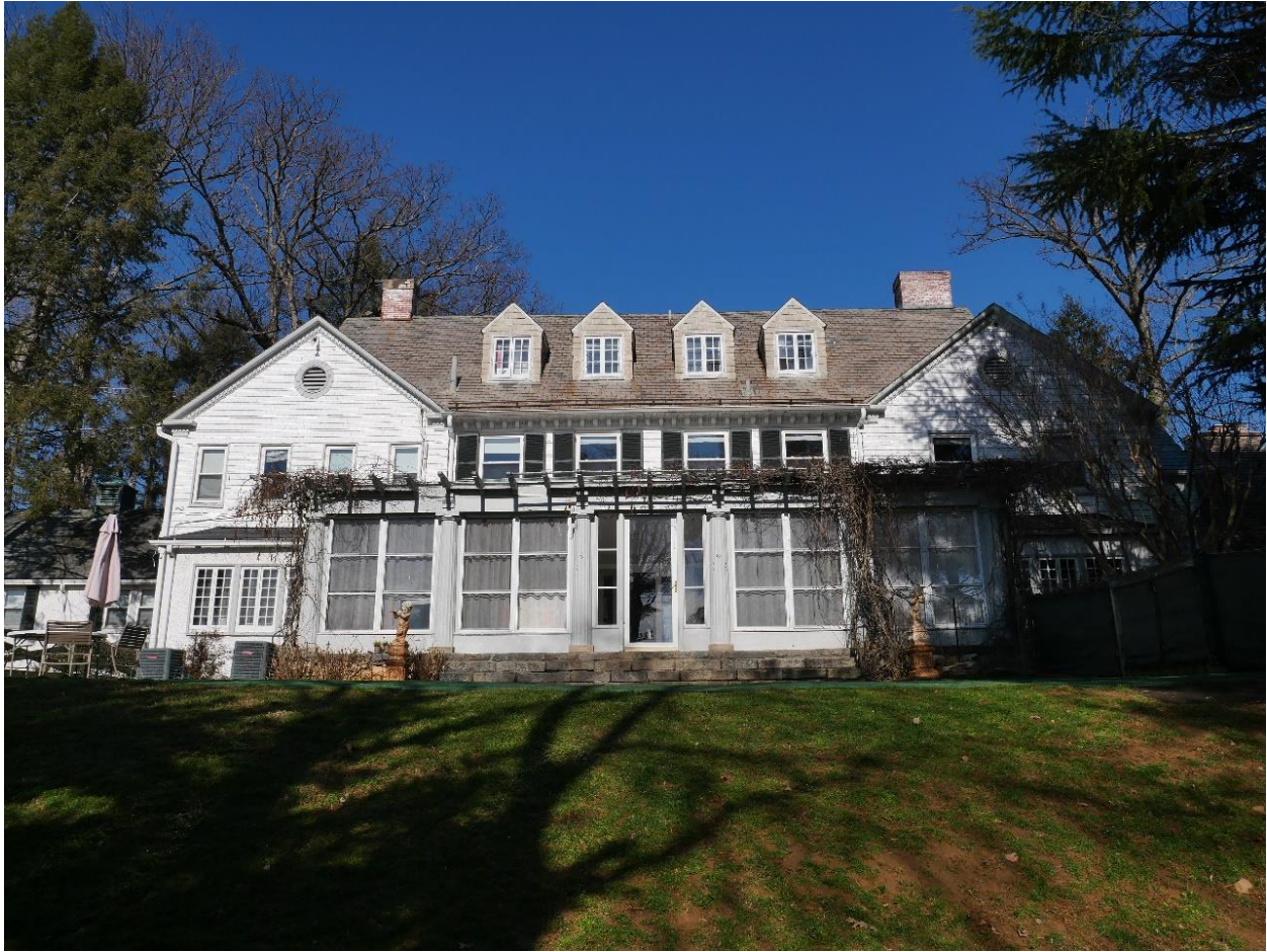
Figure 6: View of the south elevation of the 1901 dwelling, 2022. Source: Historic Preservation Office, Montgomery Planning.
