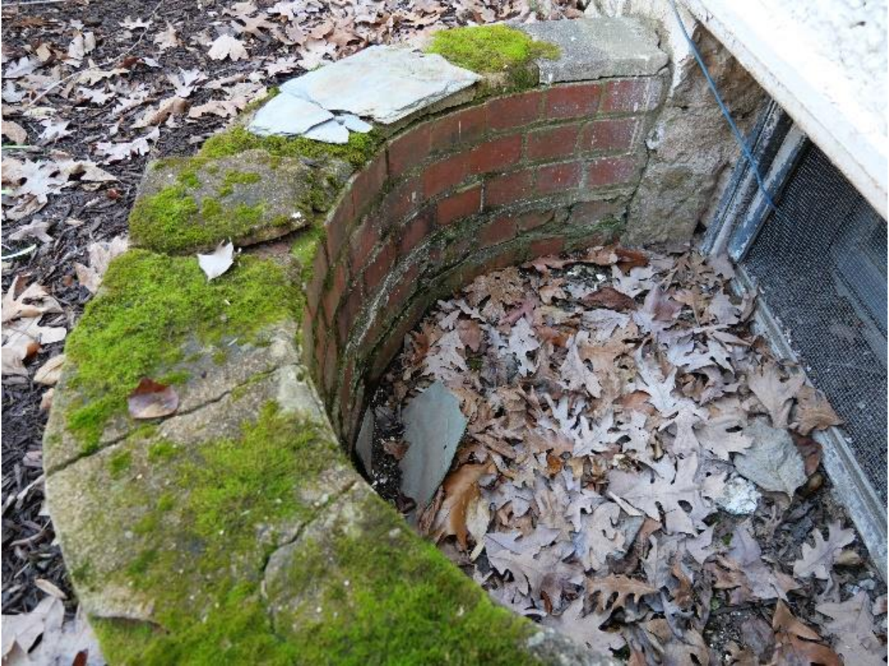
Figure 16: Detail of window well on north elevation of 1901 home, 2022. Source: Historic Preservation Office, Montgomery Planning.
