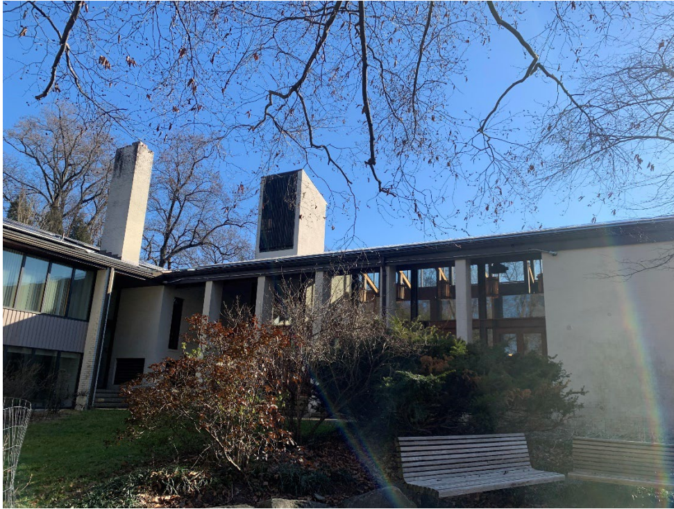
MD_Montgomery County_River Road Unitarian Church_0008 West elevation of sanctuary (Davenport January 2024)
