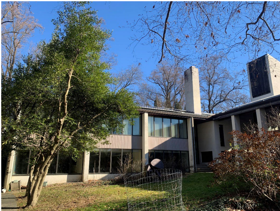
MD_Montgomery County_River Road Unitarian Church_0009 South elevation of the classroom and office wing (Davenport January 2024)
