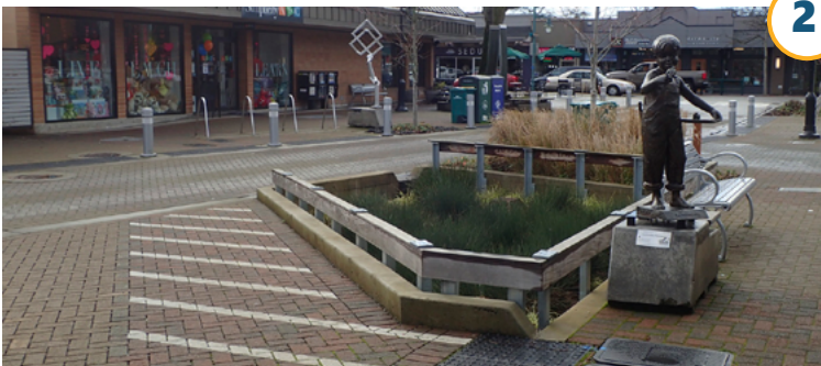
Figure 42. Example of a Bioretention on a Curbless Street in Kirkland, WA
