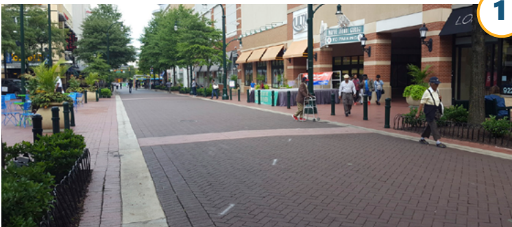
Figure 41. Example of a Valley Gutter on a Curbless Street in Silver Spring, MD
