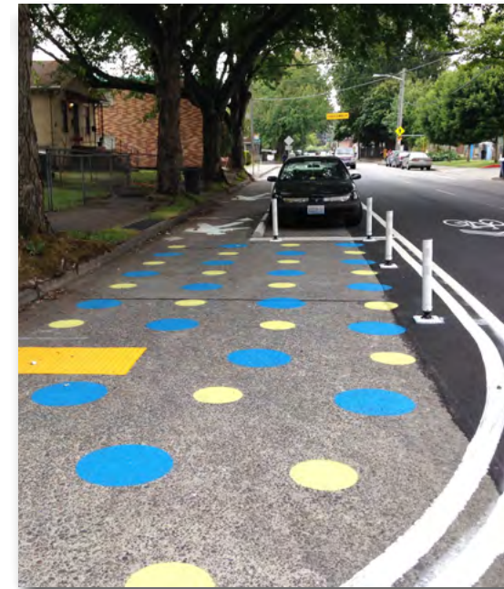
A painted pedestrian pathway in the street is separated from traffic by parked cars, temporary concrete curbs, and white flex posts. Photo Credit: Dongho Chang
