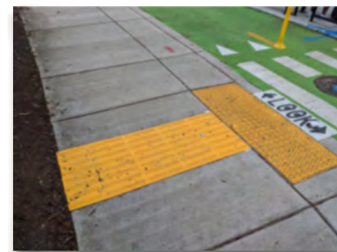
Example of a TWSI used in Montgomery County to direct people with vision disabilities to a floating bus stop
