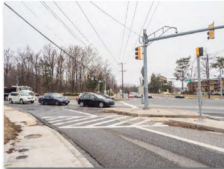
A channelized right turn lane with porkchop island at Bel Pre Road and Georgia Avenue is difficult to navigate.
