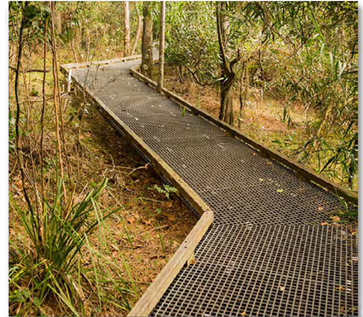
A metal boardwalk snakes through parkland. Image Credit: Marco Specialty Steel
