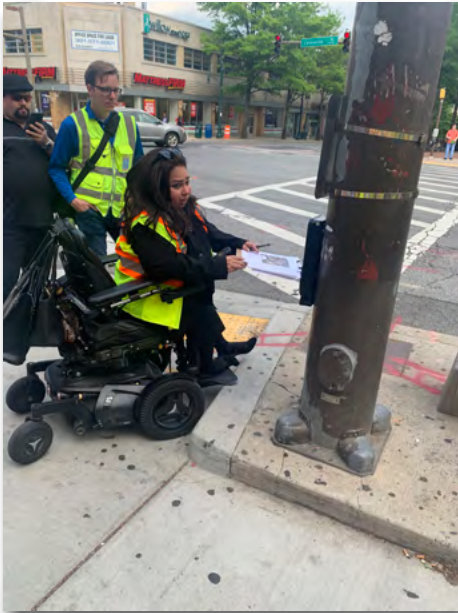
This pedestrian is unable to reach an APS in Downtown Silver Spring because the push button is located on a raised surface that her mobility device cannot navigate.
