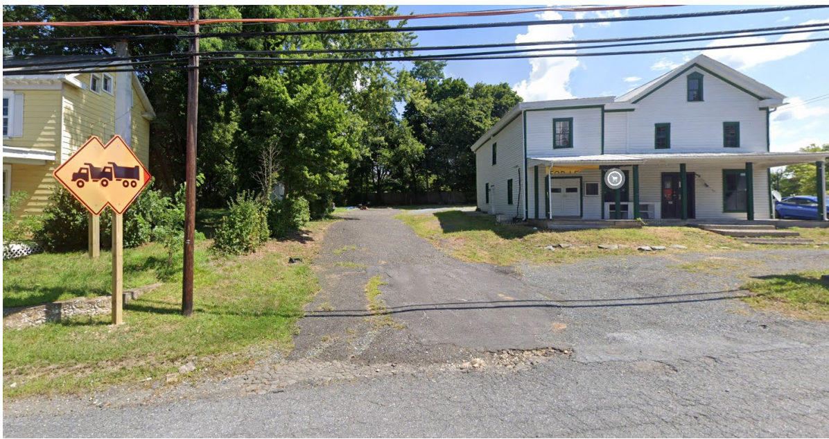
Figure 3: The subject property is located between the circa 1860 building at 23345 Frederick Road to the west (left), and the circa 1842 building to the east (right) at 23341 Frederick Road. Source: Google
