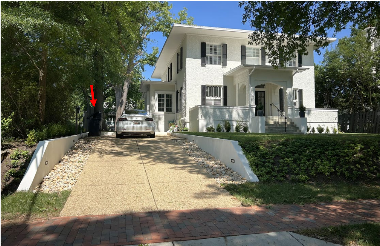
Figure 4: Front (south) elevation of the subject property. The red arrow denotes the approximate location of the proposed enclosure.
