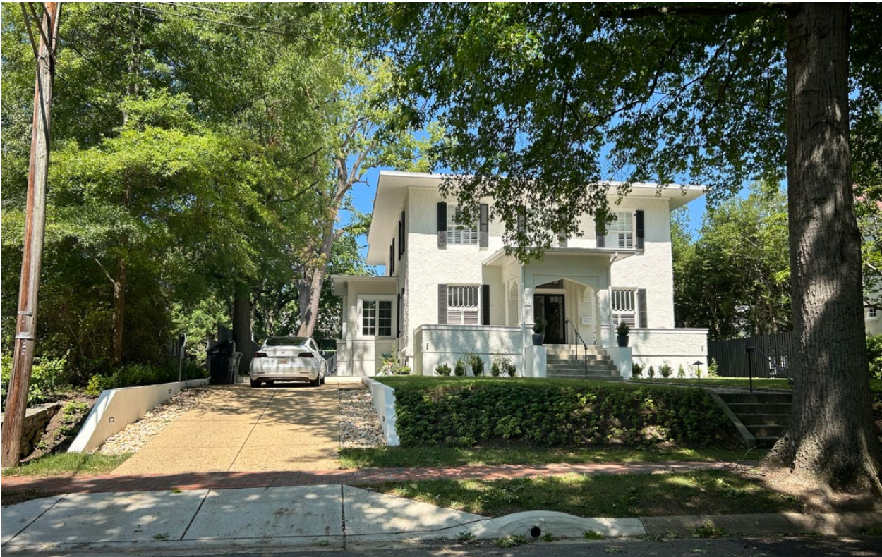
Figure 8: Front elevation of 13 Grafton Street. The proposed enclosure would be located along the western property line (left), immediately beyond the existing driveway.
