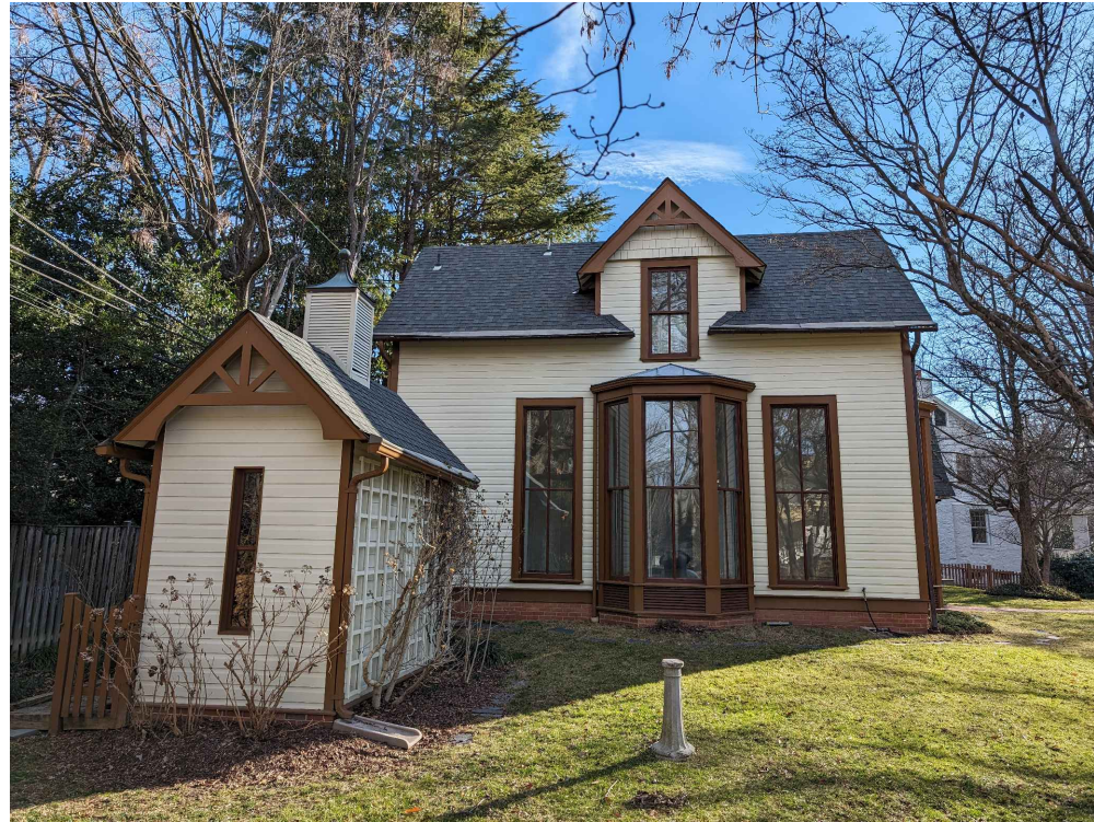
LEFT SIDE VIEW W/ SHED
