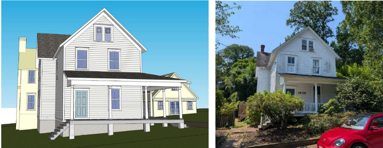
Figure 3: A secondary corbelled chimney is visible on the east elevation of the existing building (right), but not shown on the drawings or renderings in the submission. While this chimney also appears to be original, it is not as character-defining of the property as the larger chimney on the west elevation.
