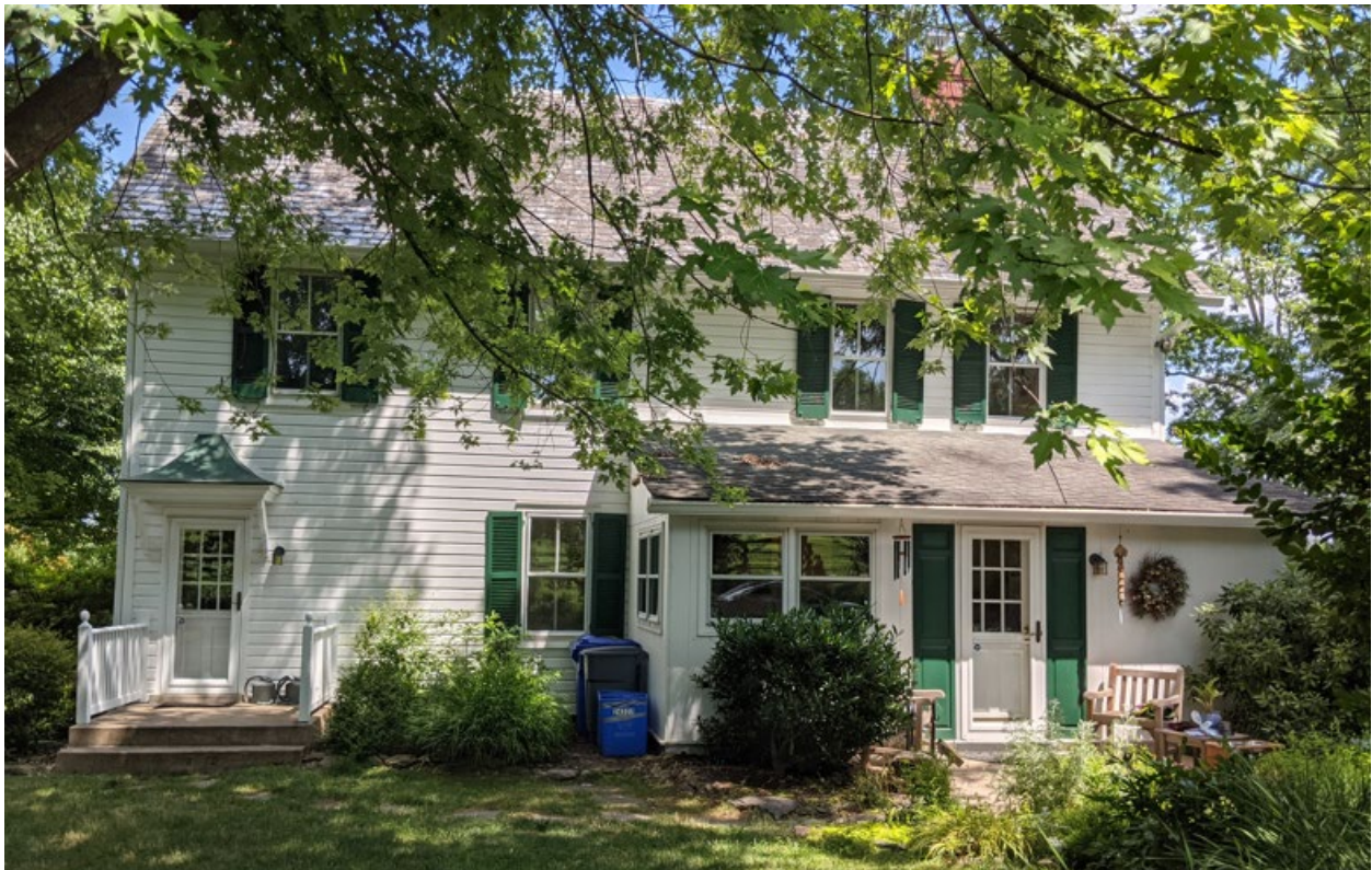
Figure 5: West elevation showing the non-historic shed roof addition.
