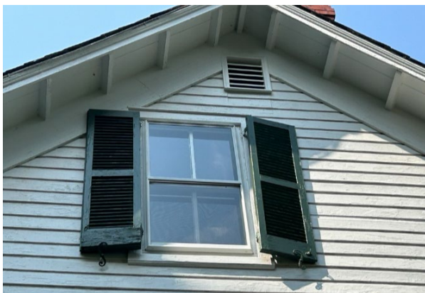
Figure 10: Detail of existing window on south gable end.
