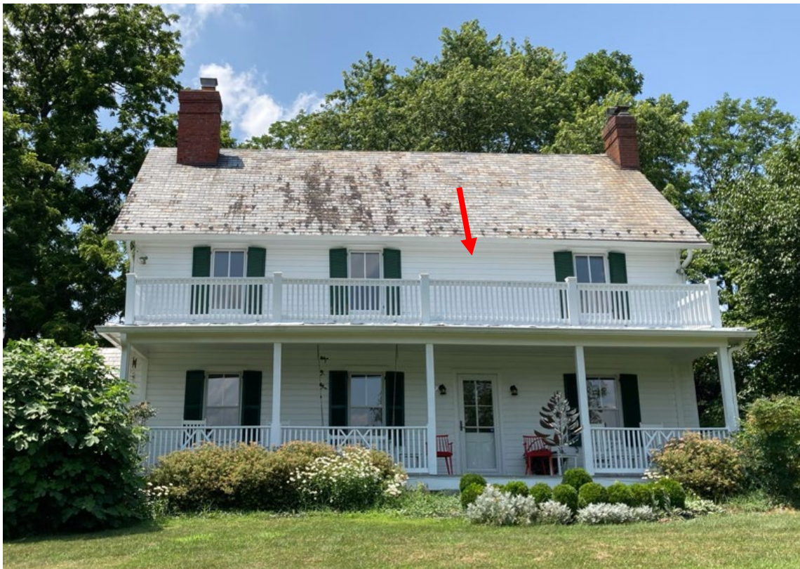
Figure 3: East elevation of the house. The red arrow points to the location of the proposed window.
