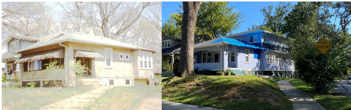
Figure 3: 7417 Baltimore Ave. before the addition (left) and after the two-story addition (right).
