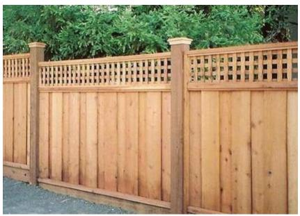
Figure 5: The applicant proposes to install a 6-foot tall board and batten fence with trellis on top in the side yards.
