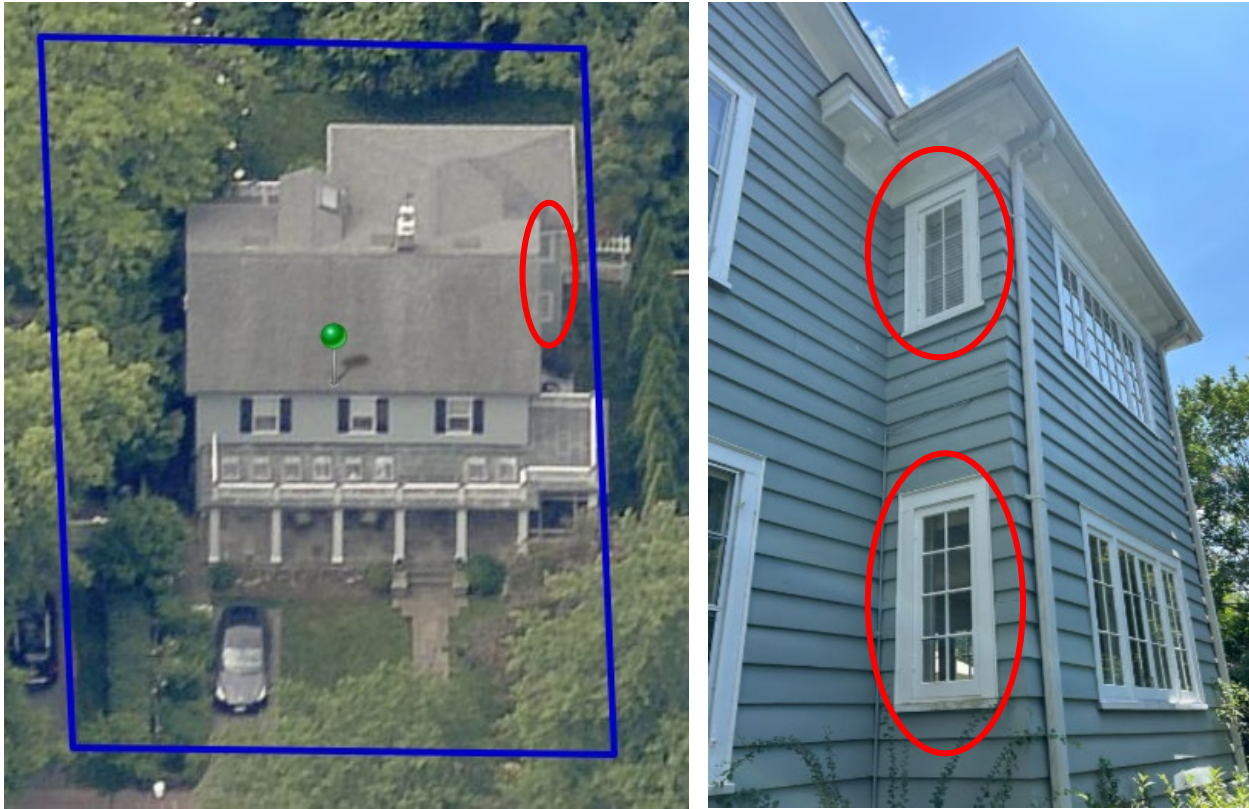
Figure 3: Area of work on the north elevation (left, circled in red), and closer view of the two north-facing windows to be replaced (right, circled in red).
