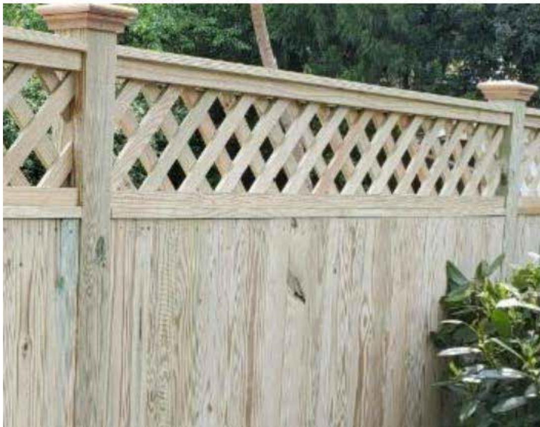
Figure 4: The applicant provided this representative photo of the fence to be installed at the subject property. It will stand 6 feet, 4 inches, tall with a 5-foot tall solid board base, 1-foot tall lattice top, and 4-inch tall post caps.
