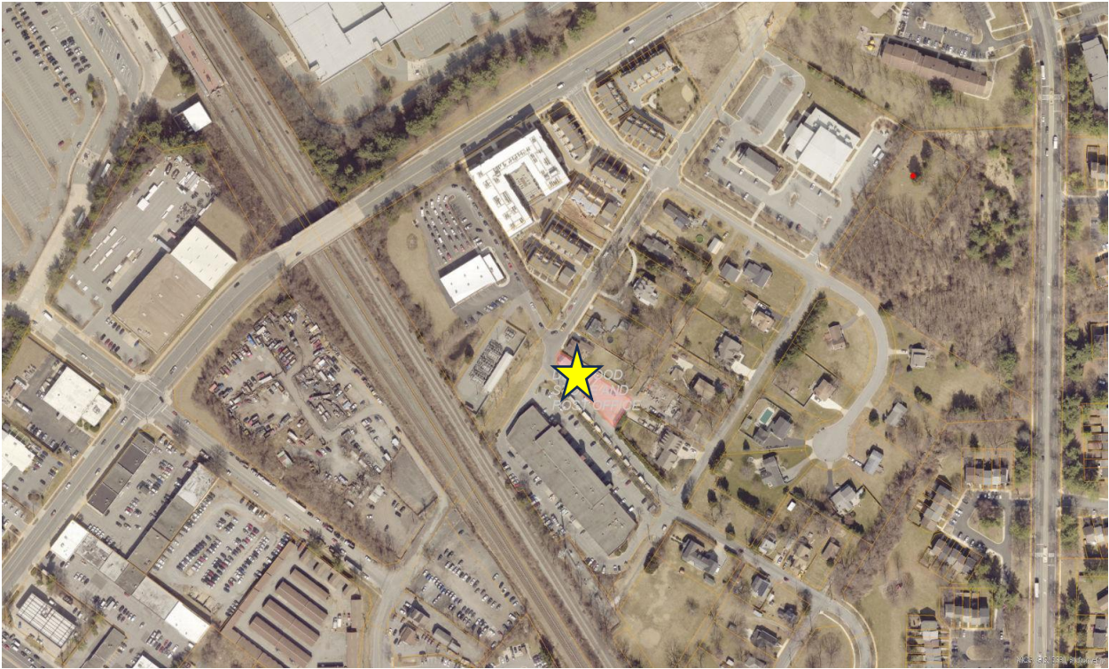
Figure 1: The Derwood Store and Post Office is located at the corner of Redland Rd. and Chieftain Ave.
