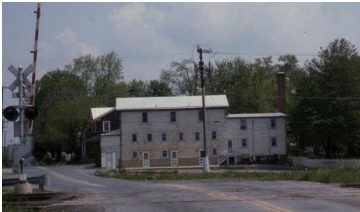
Figure 7: Photo of the subject property from 1975.
