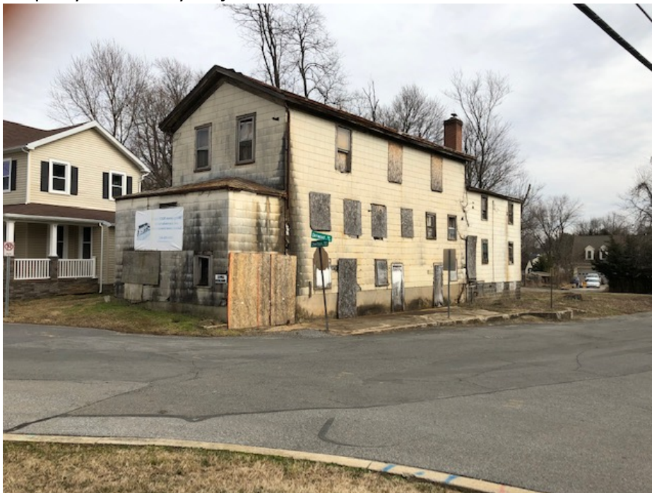
Property before any major work started
