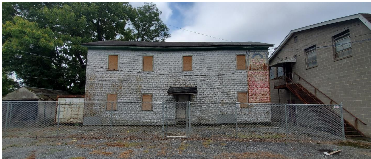
Figure 4: View of the facade of Hoyle's Mill, 2023.
