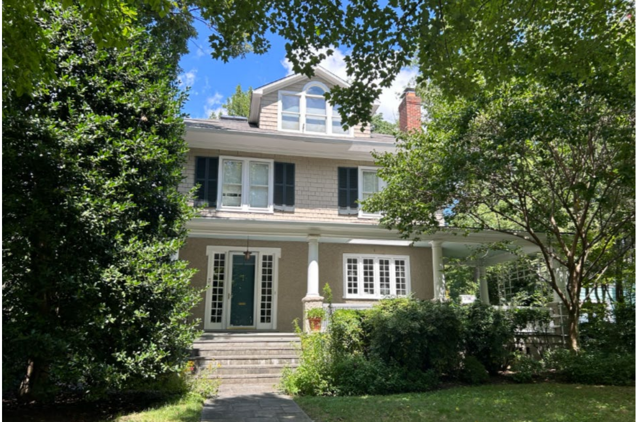
Figure 2: Front (south) elevation of 3 Hesketh Street, August 2024 (Historic Preservation Office).
