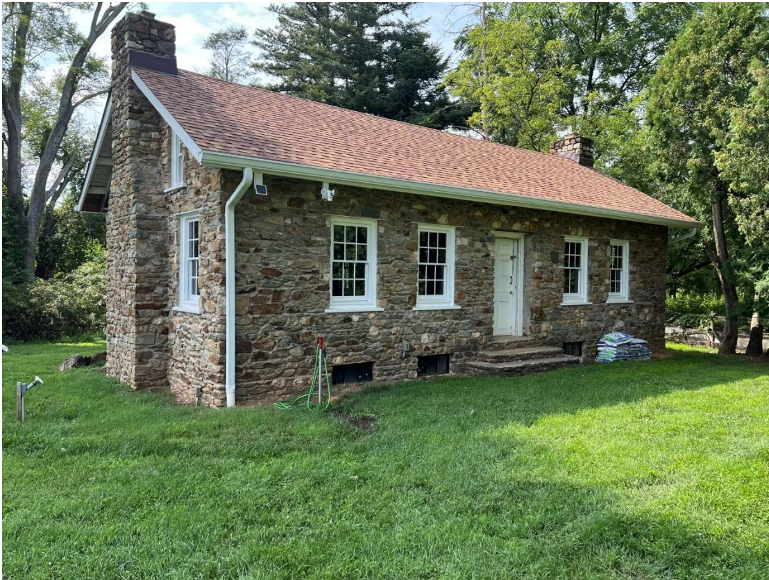
Figure 1. Front/side elevation view of stone cottage
