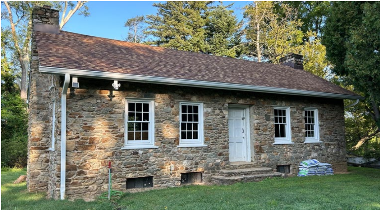
Figure 2: The stone tenant house, with the door proposed for replacement (center).
