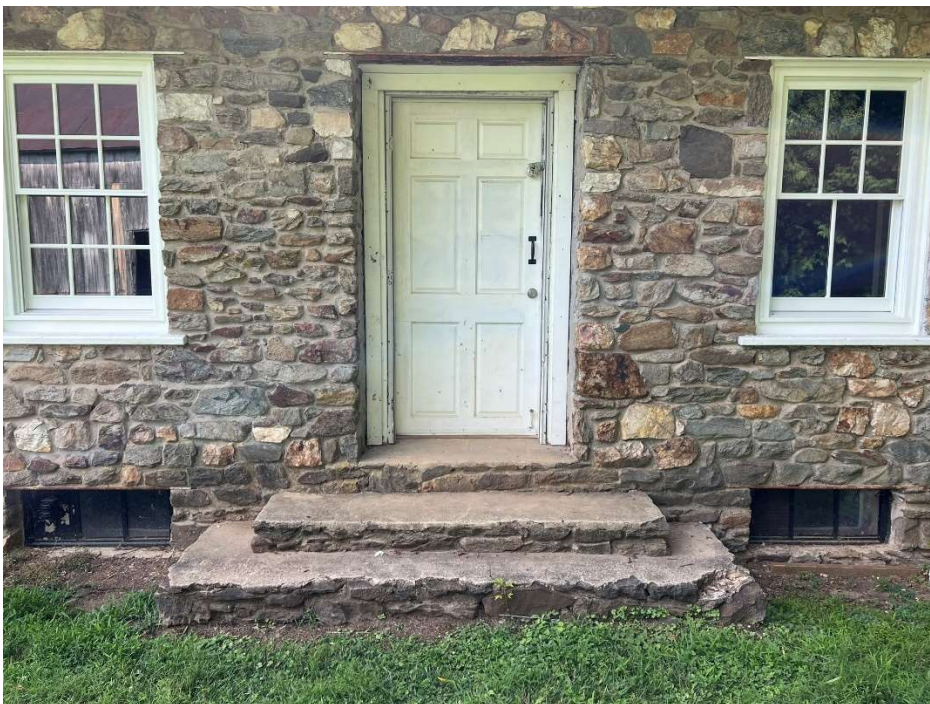
Figure 2. Existing 2014 wood door
