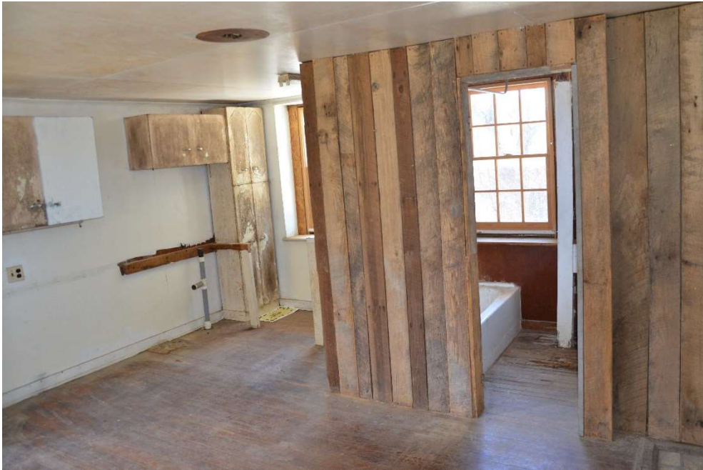
Figure 3. Sample of interior ground floor renovation work area.
