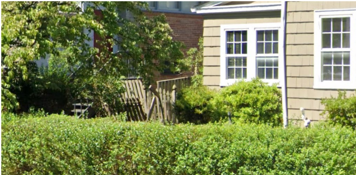
Figure 4: 2022 Google Streetview image of the 1995 fence that was replaced. As evident in the image, this portion of the fence was falling down.
