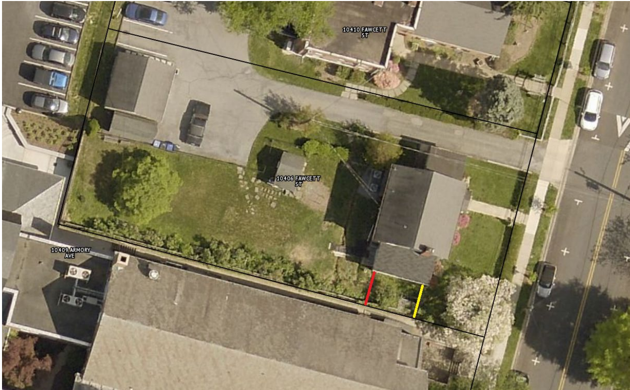
Figure 5: Location of previous fence installed in 1995 (in yellow) and new fence installed in 2024 (in red).
