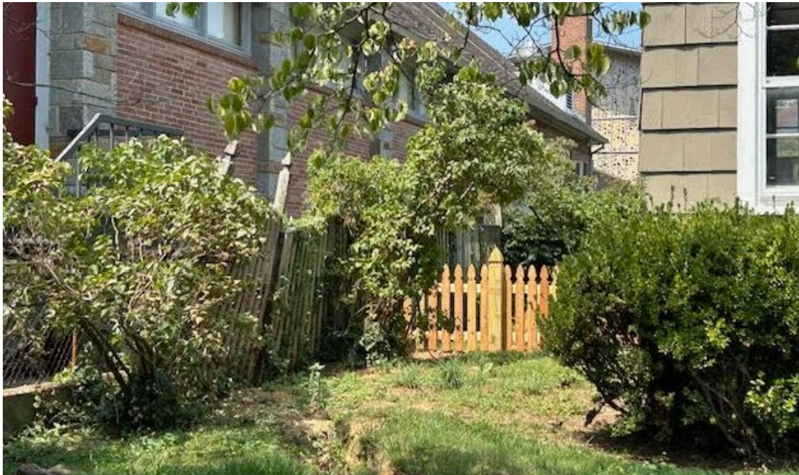
Figure 3: The newly-installed fence, August 2024 (Historic Preservation Office).
