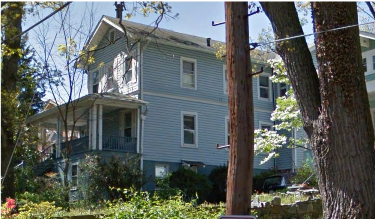
Figure 5: The front (southeast) and right side (northeast) elevations of 36 Columbia Ave.
