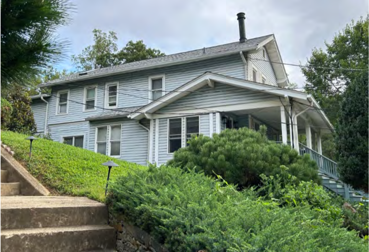
Figure 4: The left (southwest) side elevation of 36 Columbia Ave.
