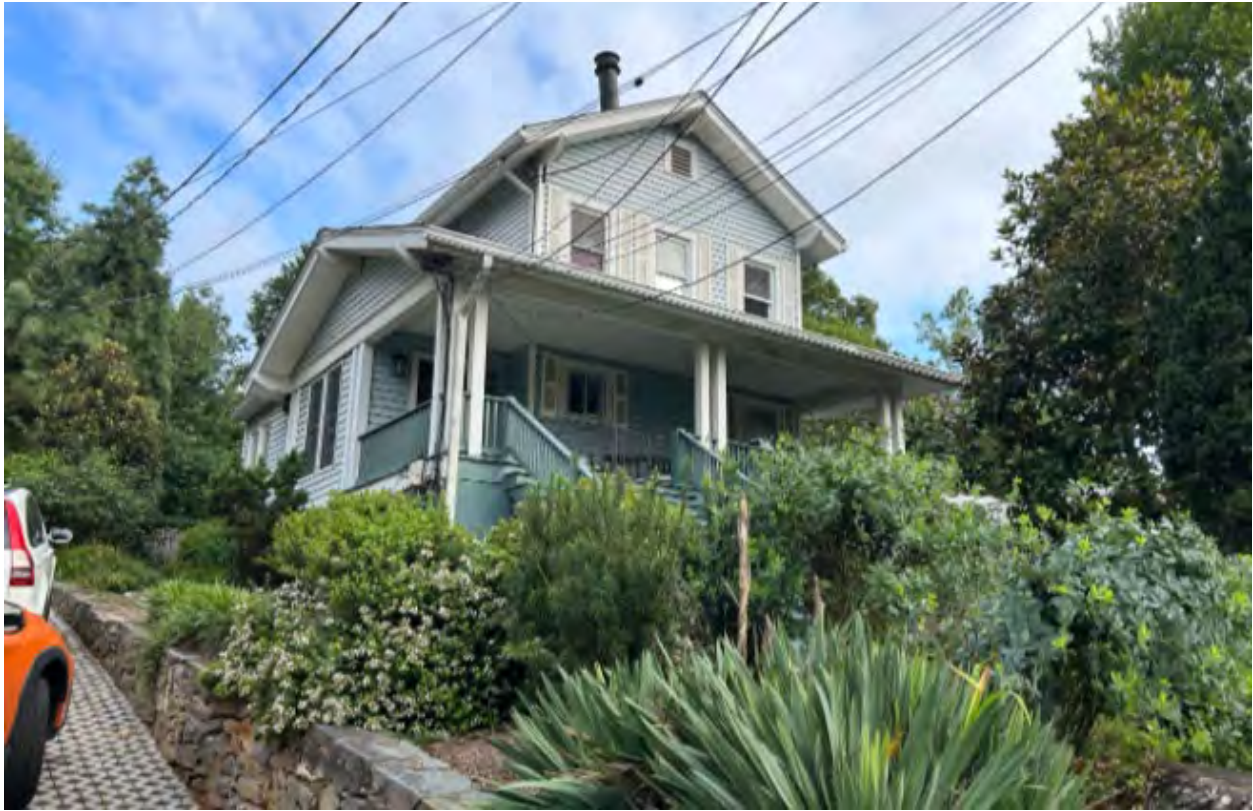
Figure 2: The front (southeast) elevation of 36 Columbia Ave. from the sidewalk in front of the house.
