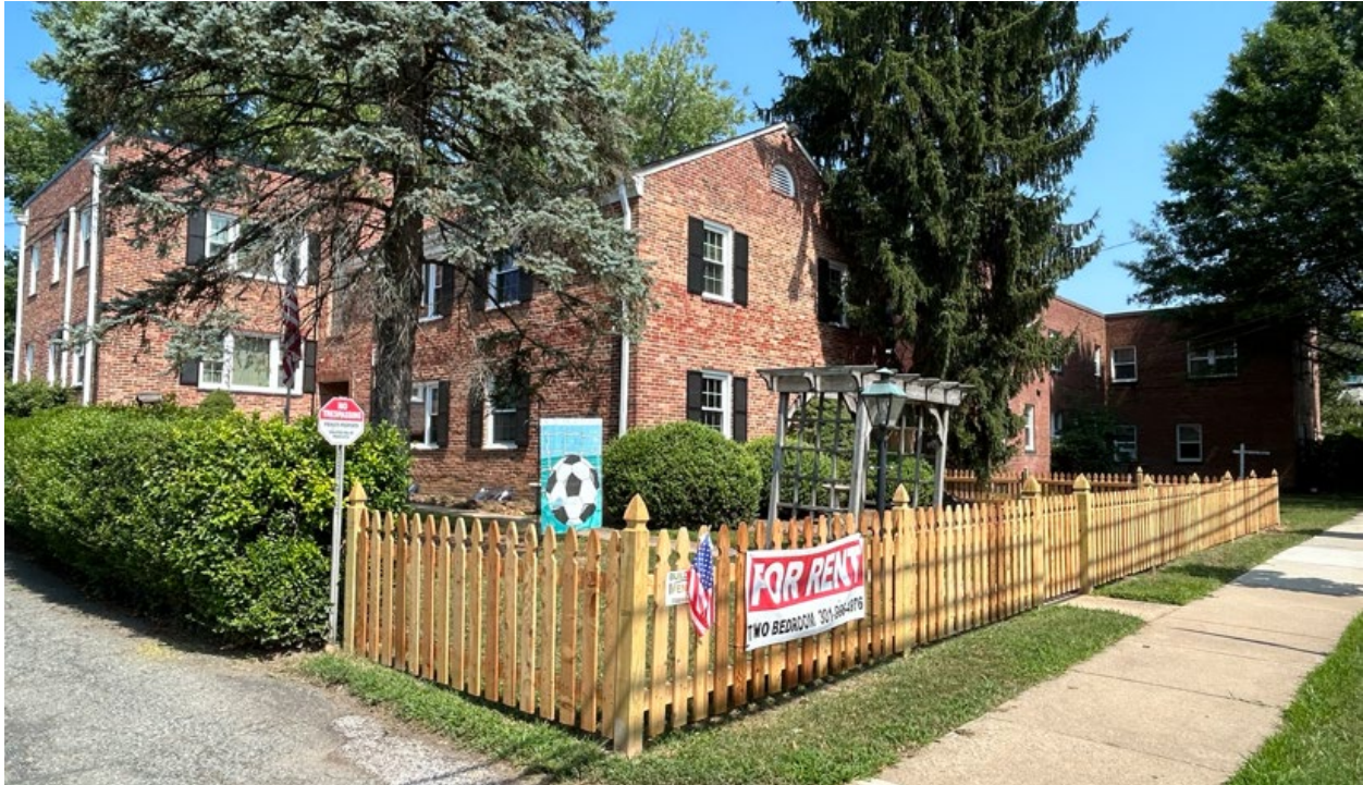
Figure 2: View of the front elevation of 10410 Fawcett Street with recently-installed wood fencing in the foreground, July 2024 (Historic Preservation Office).
