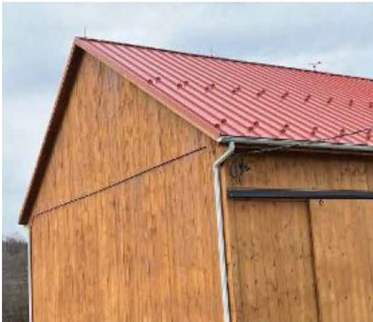
Figure 6: The standing-seam metal roof on the barn is recently installed.
