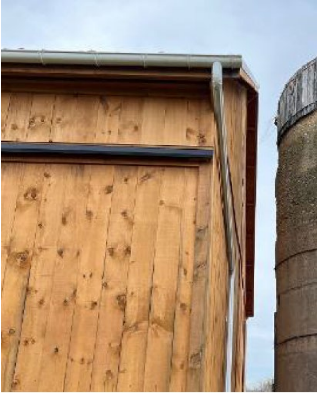
Right Side of Structure
