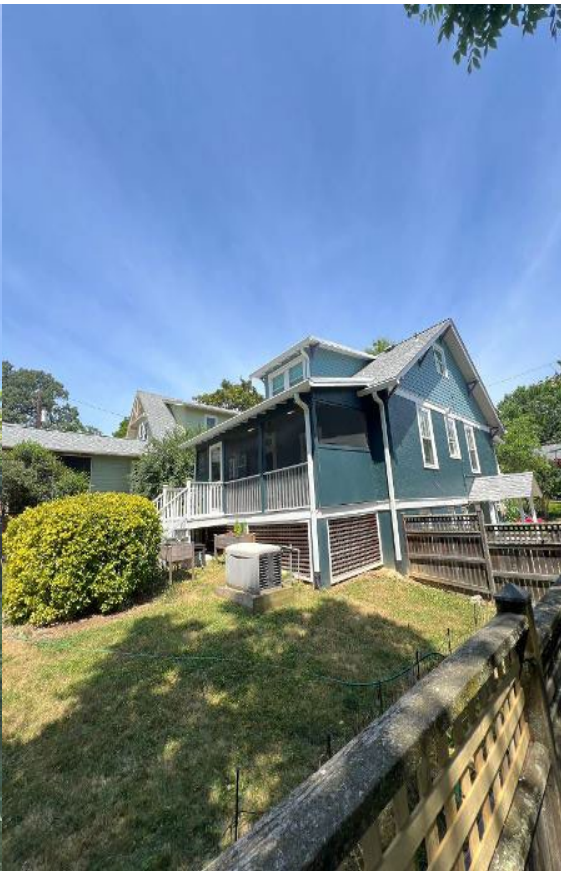
Rear Side of House
