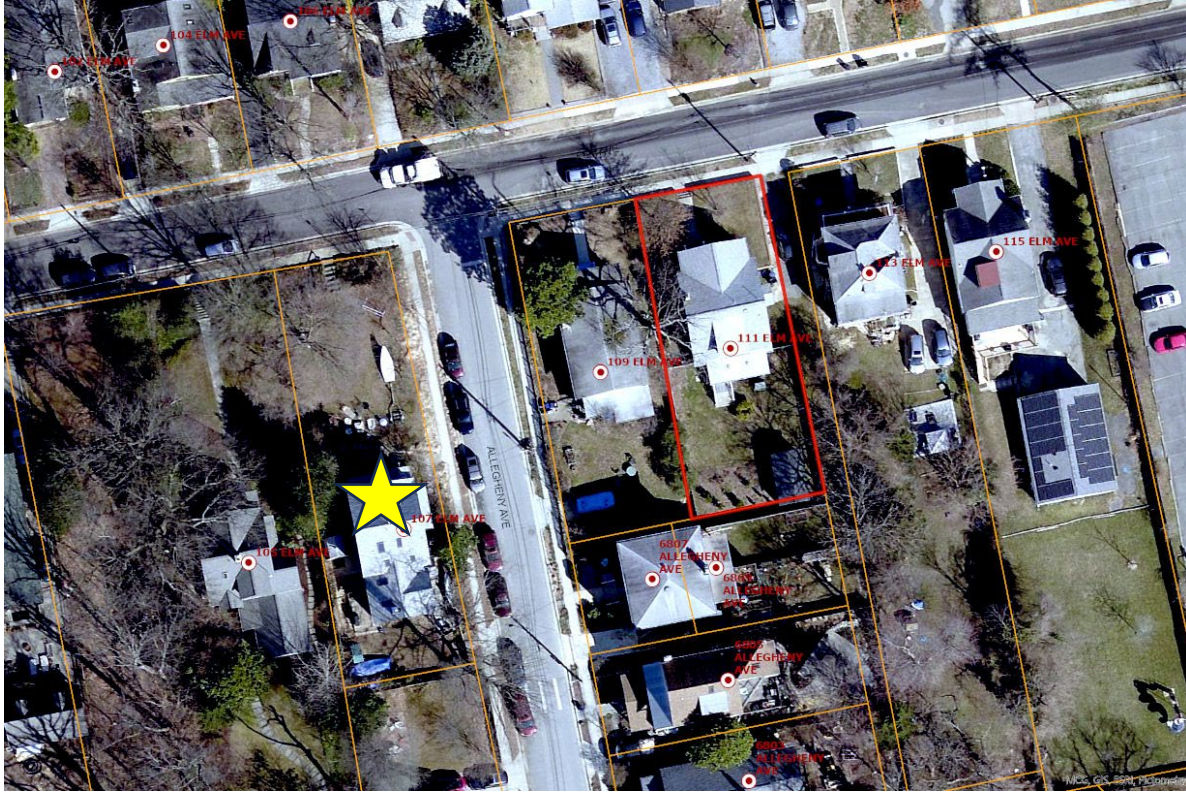
Figure 7: The subject property is outlined in red. The starred Outstanding Resource at 107 Elm Ave. is located approximately 125 feet away and within the viewshed.
