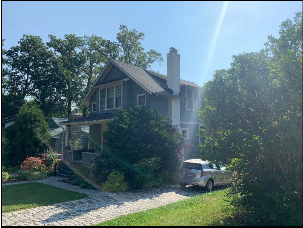
Figure 3: The front and right-side elevations of 7209 Willow Ave.
