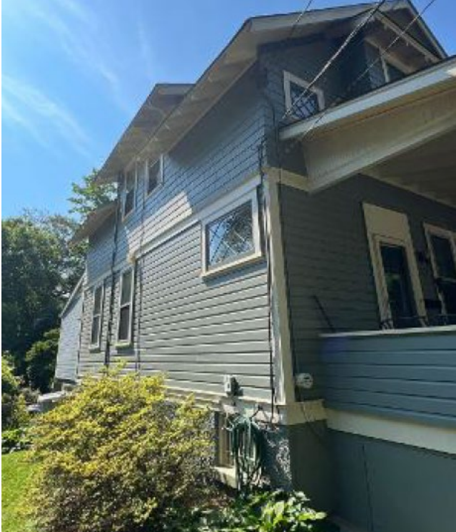
Before Utility Install
