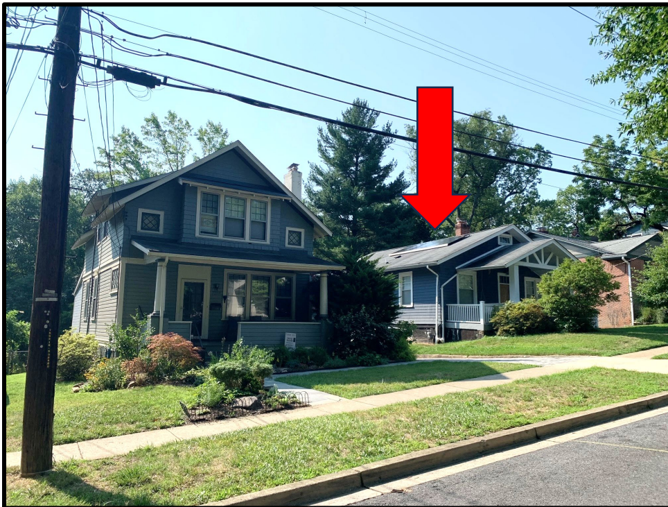
Figure 6: The HPC approved solar panels on the adjacent Contributing Resource at 7207 Willow Avenue (indicated with a red arrow) at the November 15, 2023, meeting. The subject property at 7209 Willow Avenue is in the foreground.
