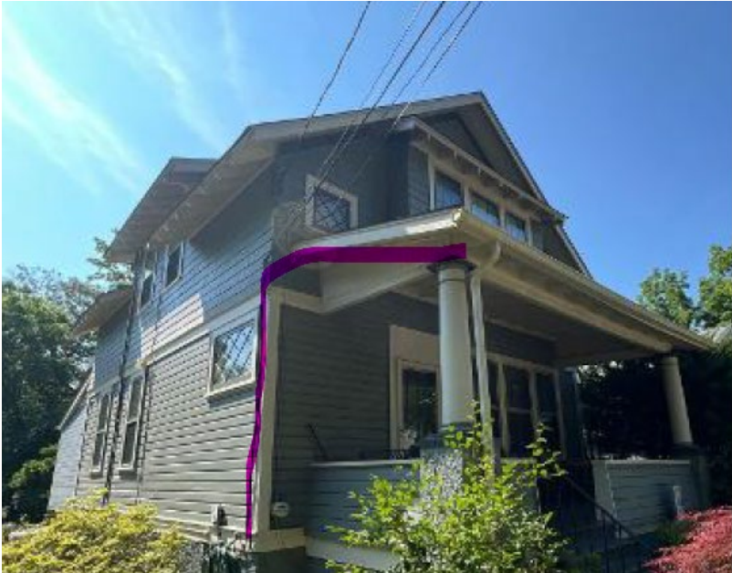
After Utility Install
