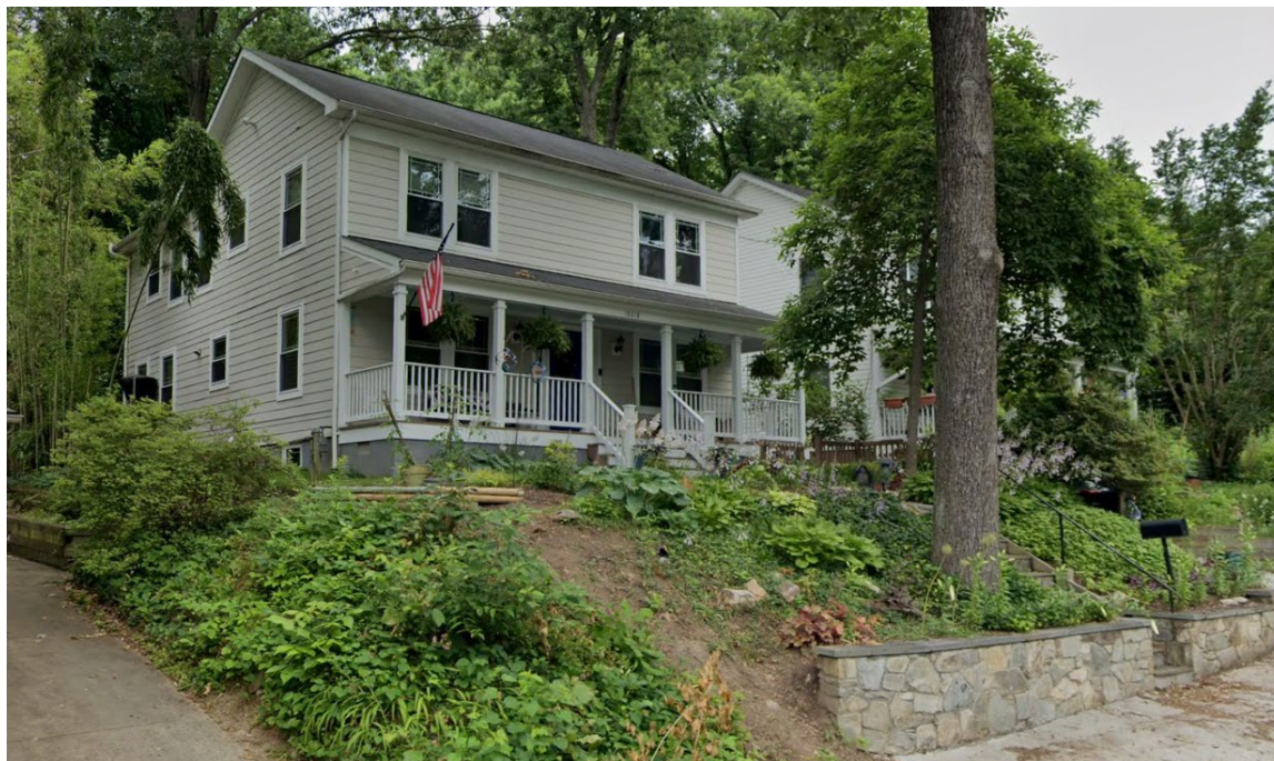
Figure 2: This Google Streetview image shows the existing building in 2022. The proposed work would take place at the base of the porch and the front steps leading to the porch.
