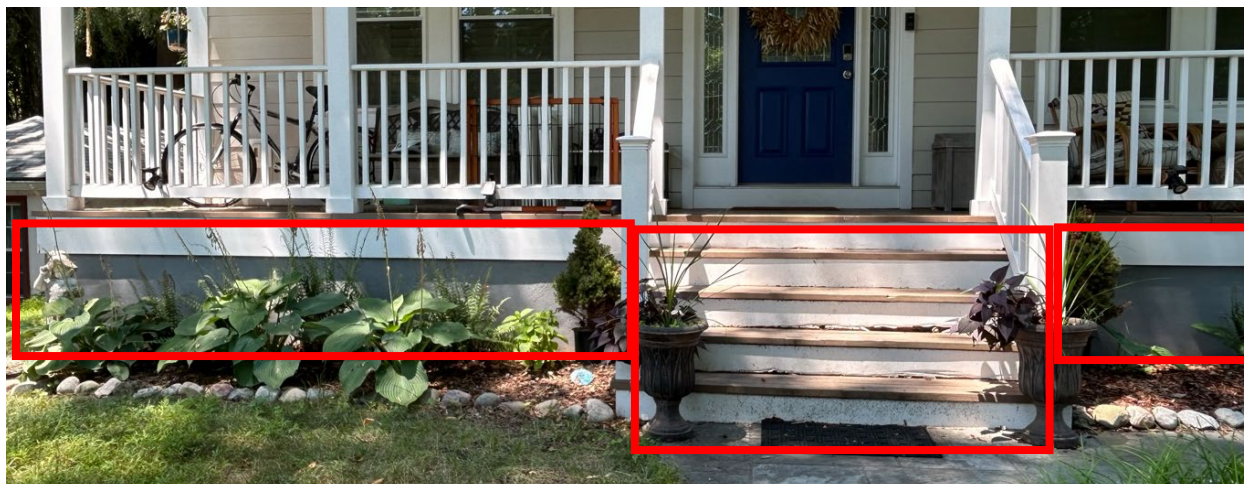
Figure 5: Closer view of the area of work, July 2024 (Historic Preservation Office)..
