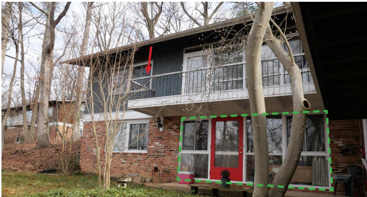
Figure 3: The south elevation of the subject house from May 2021.
