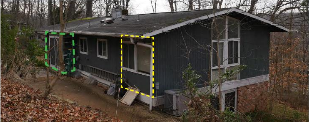
Figure 2: View of the subject house from the northwest (the green box identifies a non-historic modification).
