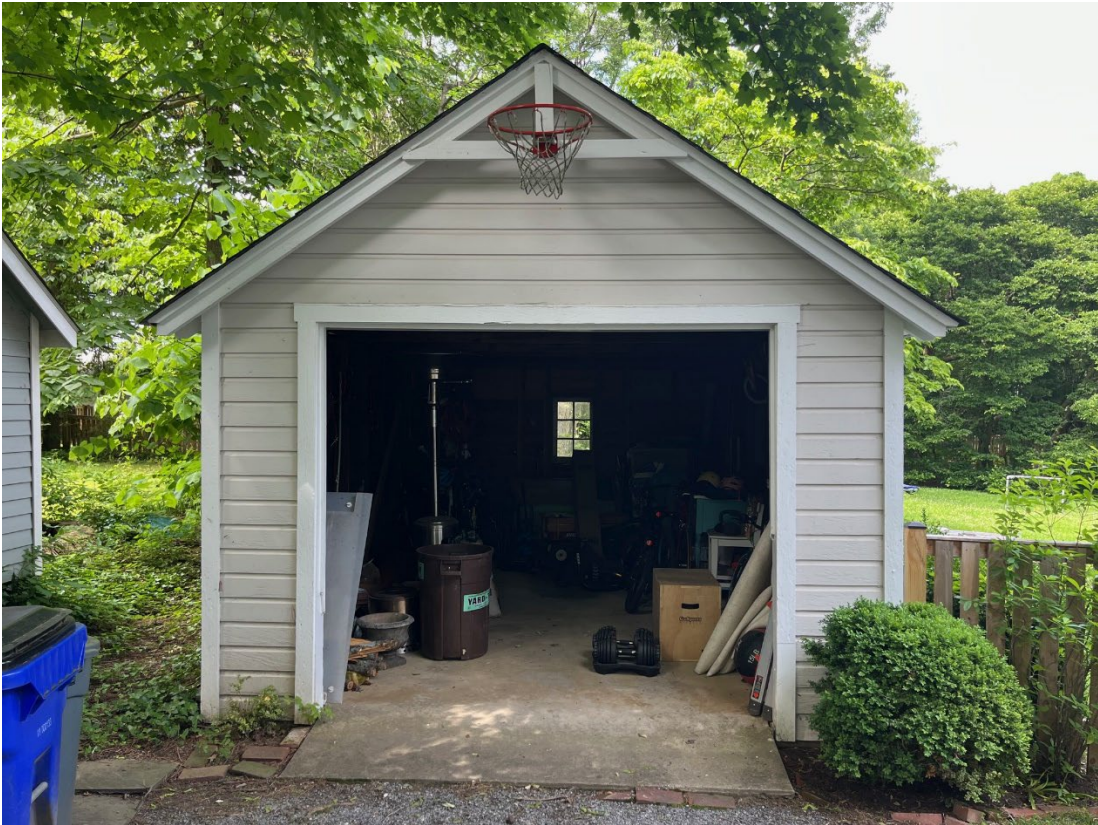
Photo 2: Front of garage, without door. Currently used for storage.
