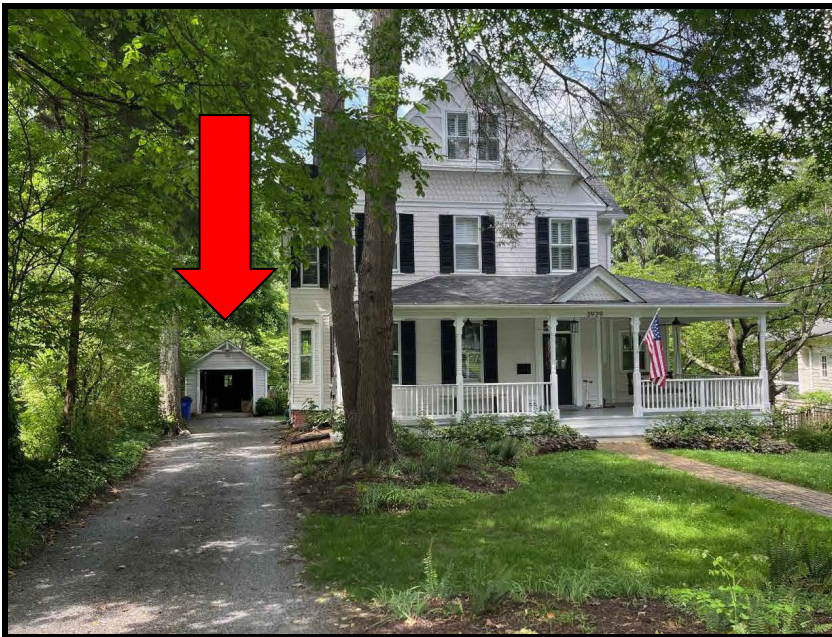
Figure 2: The applicant provided this photo of the subject property as seen from the right of way. A red arrow indicates the location of the garage.
