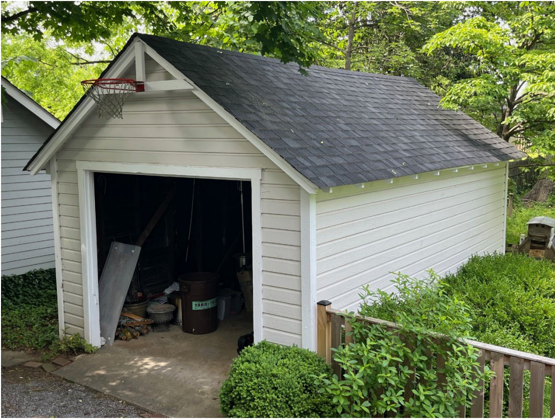
Photo 3: Front and east side of garage, from back deck.
