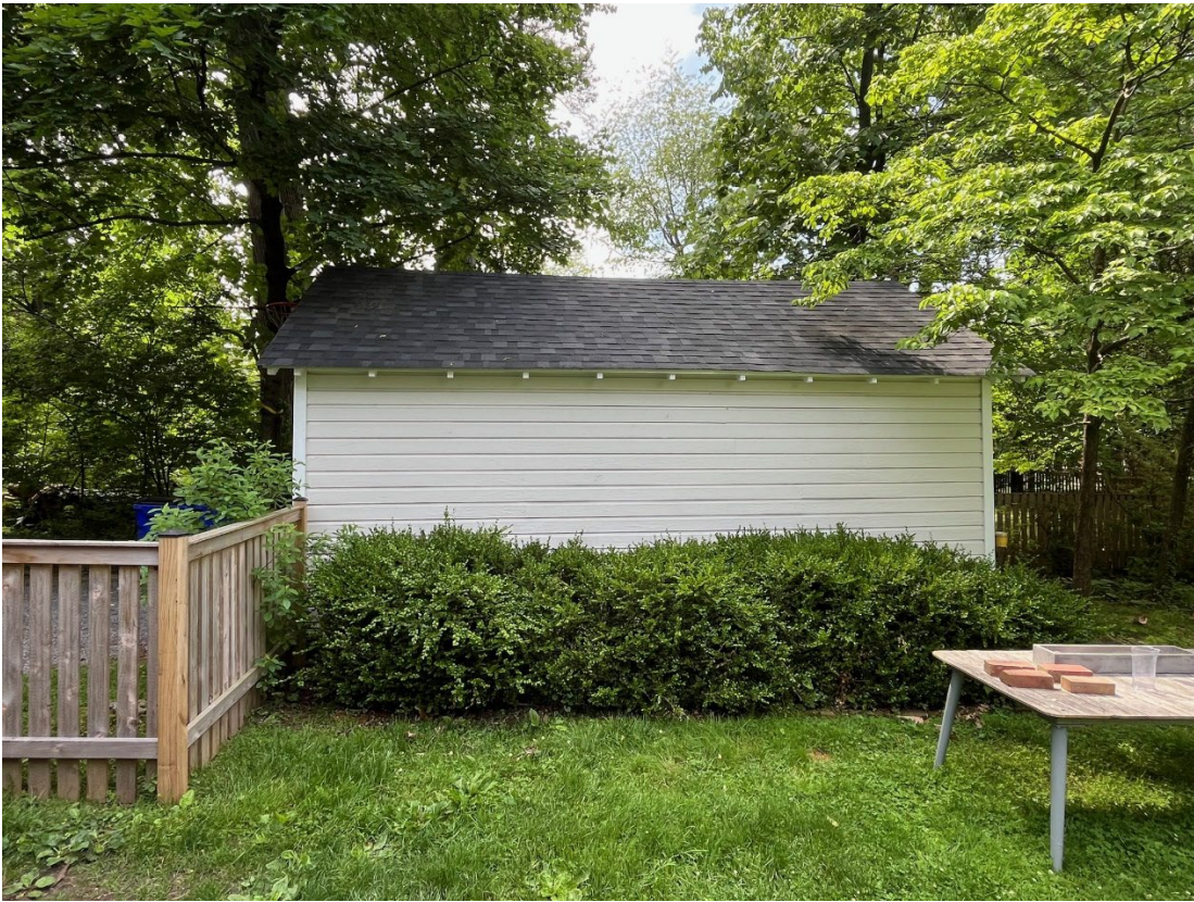
Photo 4: East side of garage, where a functional door may be added.
