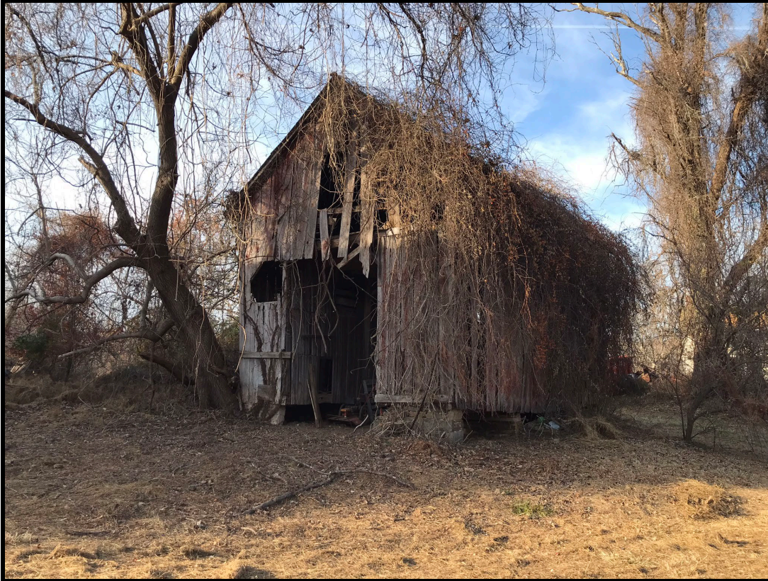
Figure 9: The rear elevation of the previous Corn Crib in 2021.
