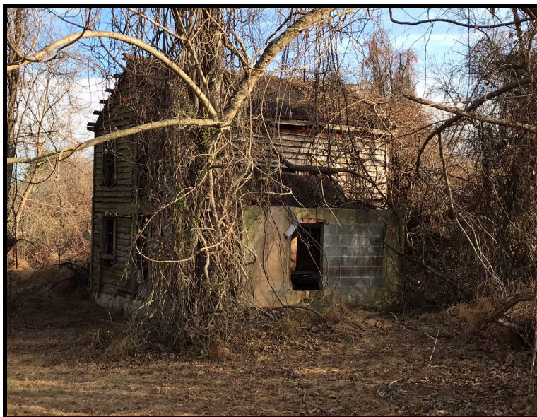
Figure 12: The front and right-side elevations of the Dairy Building in 2021.
