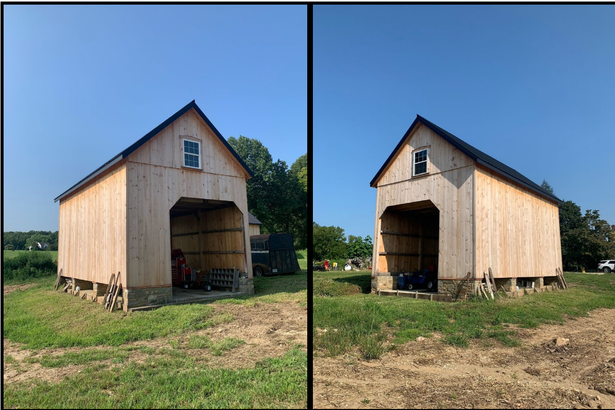
Figure 10: The front and left-side elevations of the newly constructed Corn Crib (left), and the rear and left-side elevations (right).
