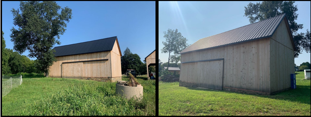
Figure 7: The front and right-side elevations of the newly constructed Hay Barn (left), and the rear and left-side elevations (right).
