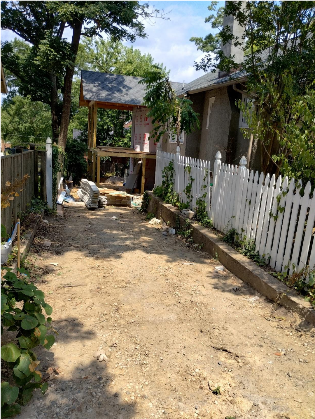
Driveway on left side of property with new construction
