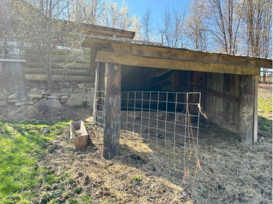
**8.) Hay Bale Shed** - For storing food for animals. This is an AG structure that has no walls, only a tin roof over repurposed telephone poles. The pictures show the stalls and then the second shows a few bales in a stall. This pavilion measures 66ft in length, 25ft in width and it is 18ft high.
