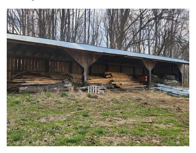
**6.) Chicken Coop** – Under construction. This coop is an AG structure. The structure is designed to be approx. 20ft high. The coop will be a 20ft square.
