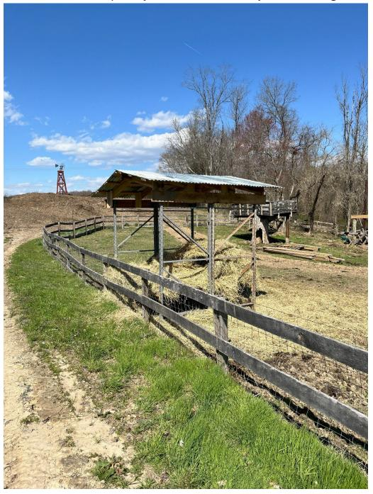
11.) Elliana Animal Feeder- Feeder for goats and sheep that is named after Jeff's other twin daughter. This feeder is in the central pasture alone. The feeder measures 8ft wide by 12ft long and stands 8ft high. This feeder is an AG structure and was also made completely from recycled materials.
