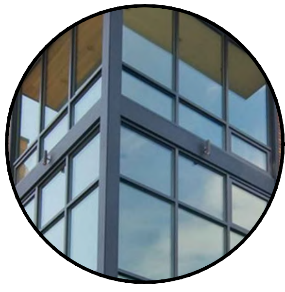
METAL PANEL AND GLAZING
