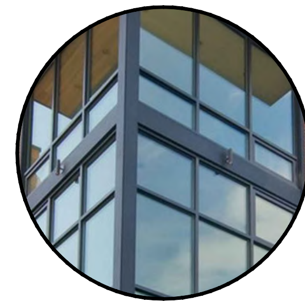
METAL PANEL AND GLAZING
