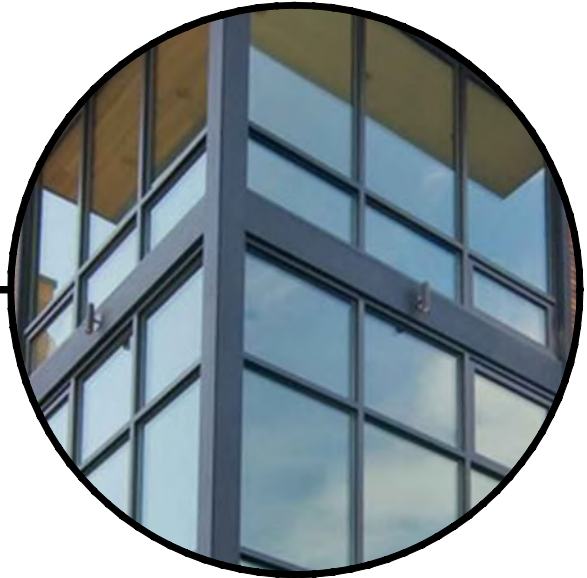
METAL PANEL AND GLAZING
