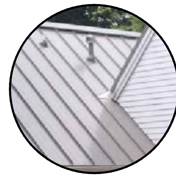
STANDING SEAM METAL ROOF
