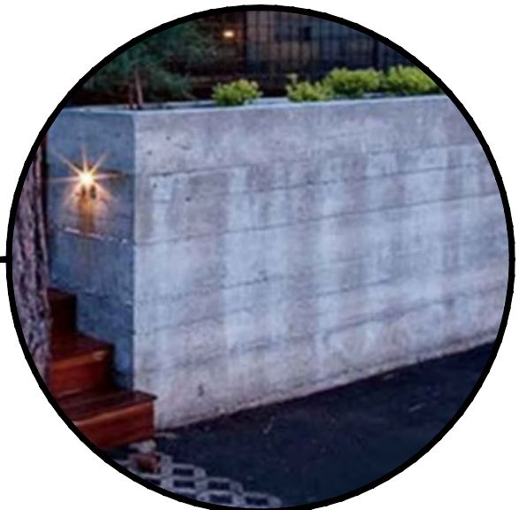
CONCRETE TERRACE WALL
