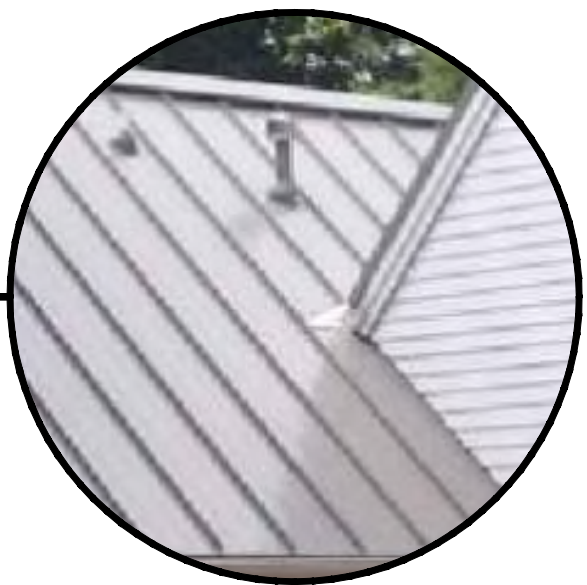
STANDING SEAM METAL ROOF
