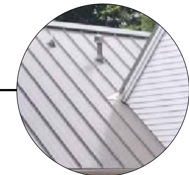
STANDING SEAM METAL ROOF
