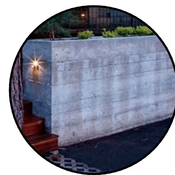
CONCRETE TERRACE WALL
