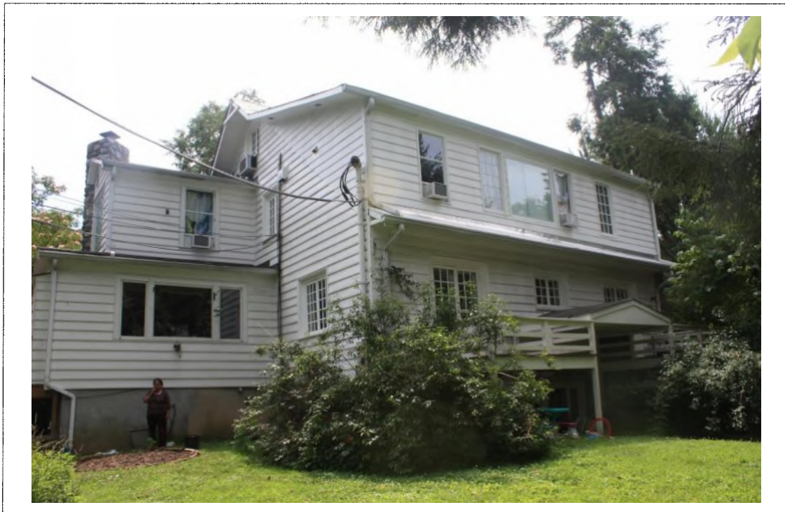
Existing West elevation. Addition to occur at this location. Dormer at second level Detail: to be reduced and original roof line at this elevation to be reconstructed.
