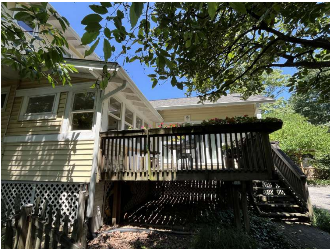
Detail: 7017 SYCAMORE AVE. SOUTH-REAR DECK CLOSE-UP
