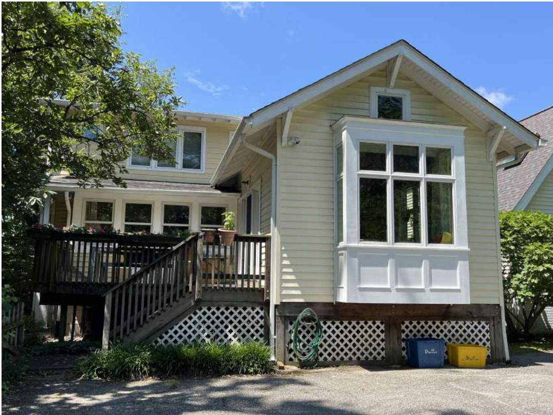
Detail: 7017 SYCAMORE AVE. REAR APPROACH
