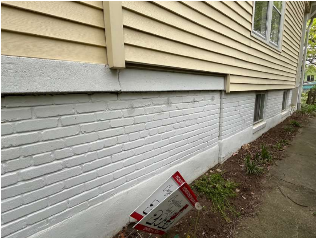
Detail: 7017 SYCAMORE AVE. FOUNDATION
